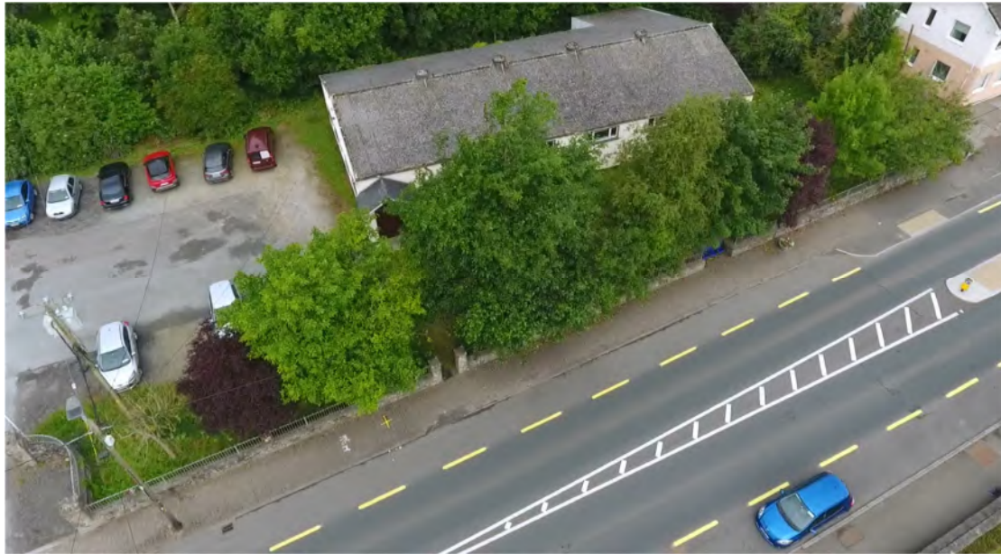
Plate 6. UAV Aerial photograph (40m elevation) at a location to the northeast of the site facing in a westerly direction showing line of trees to the East of Collon Parish Hall
