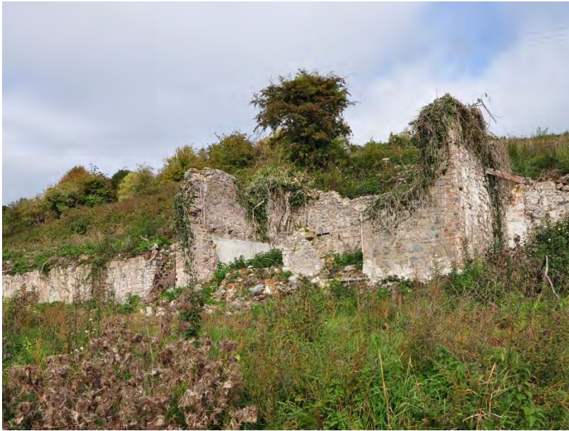
Plate 21: General view of ruined structure looking northwest.
