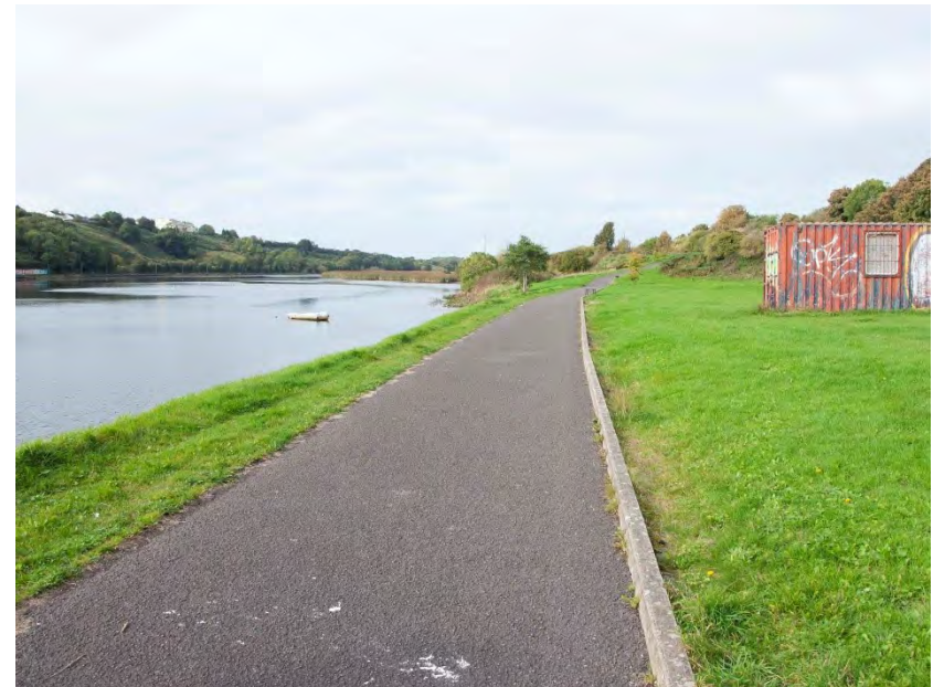
Plate 4: General view of existing path looking west.
