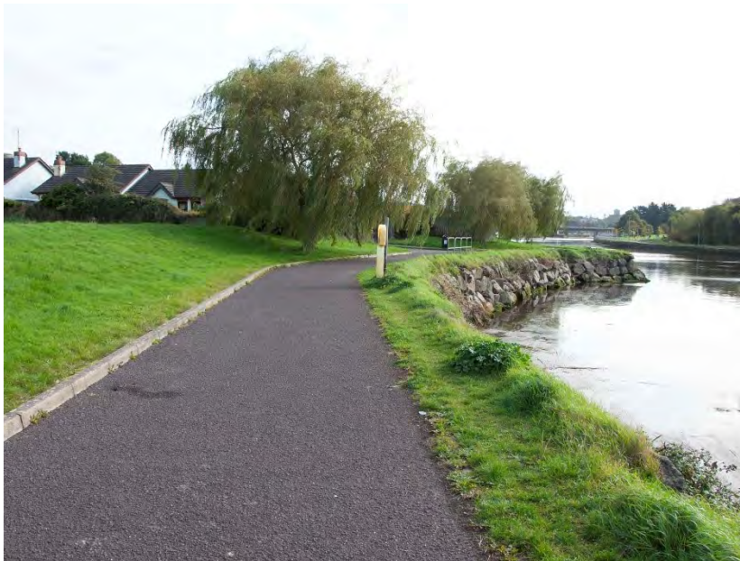
Plate 3: General view of existing path looking east towards town centre.
