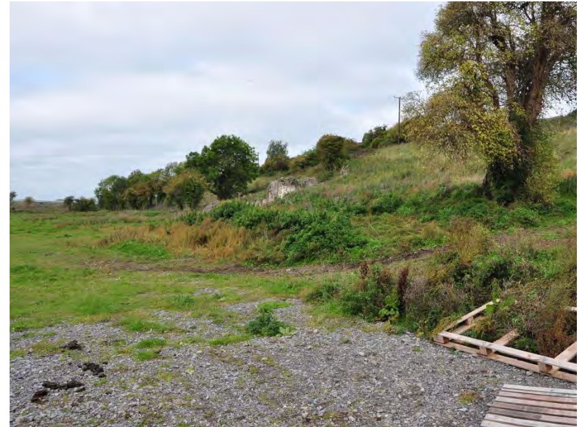
Plate 18: Existing ruined structure looking northwest.
