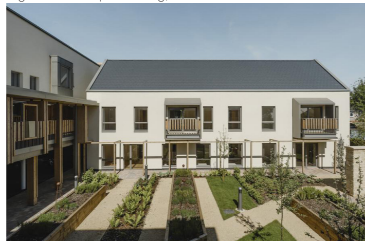
Fig.64 - Steepleton Retirement Community, Tetbury, UK.
