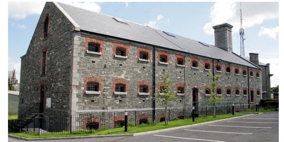
Fig.184 - Oriel Centre (former Dundalk Gaol), repair works funded by HSF.
