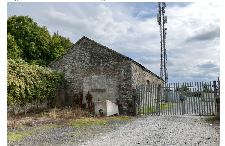
Fig.141 - View of entrance to the service yard
