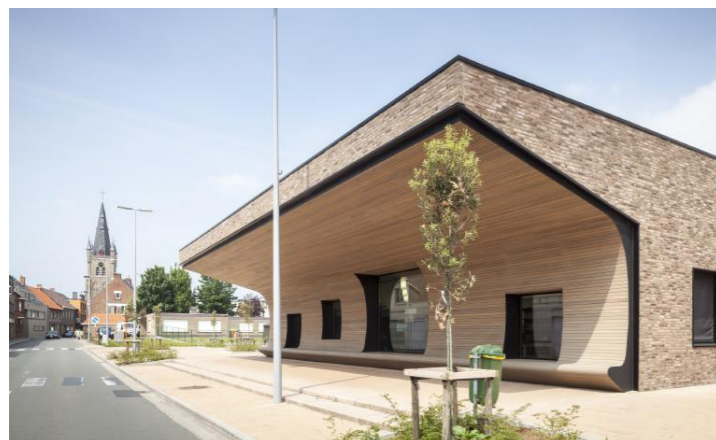
Fig.129 - Facade as public space. Cultural Centre Jonkhove, Belgium. Jozef Legrand, Dertien 12
