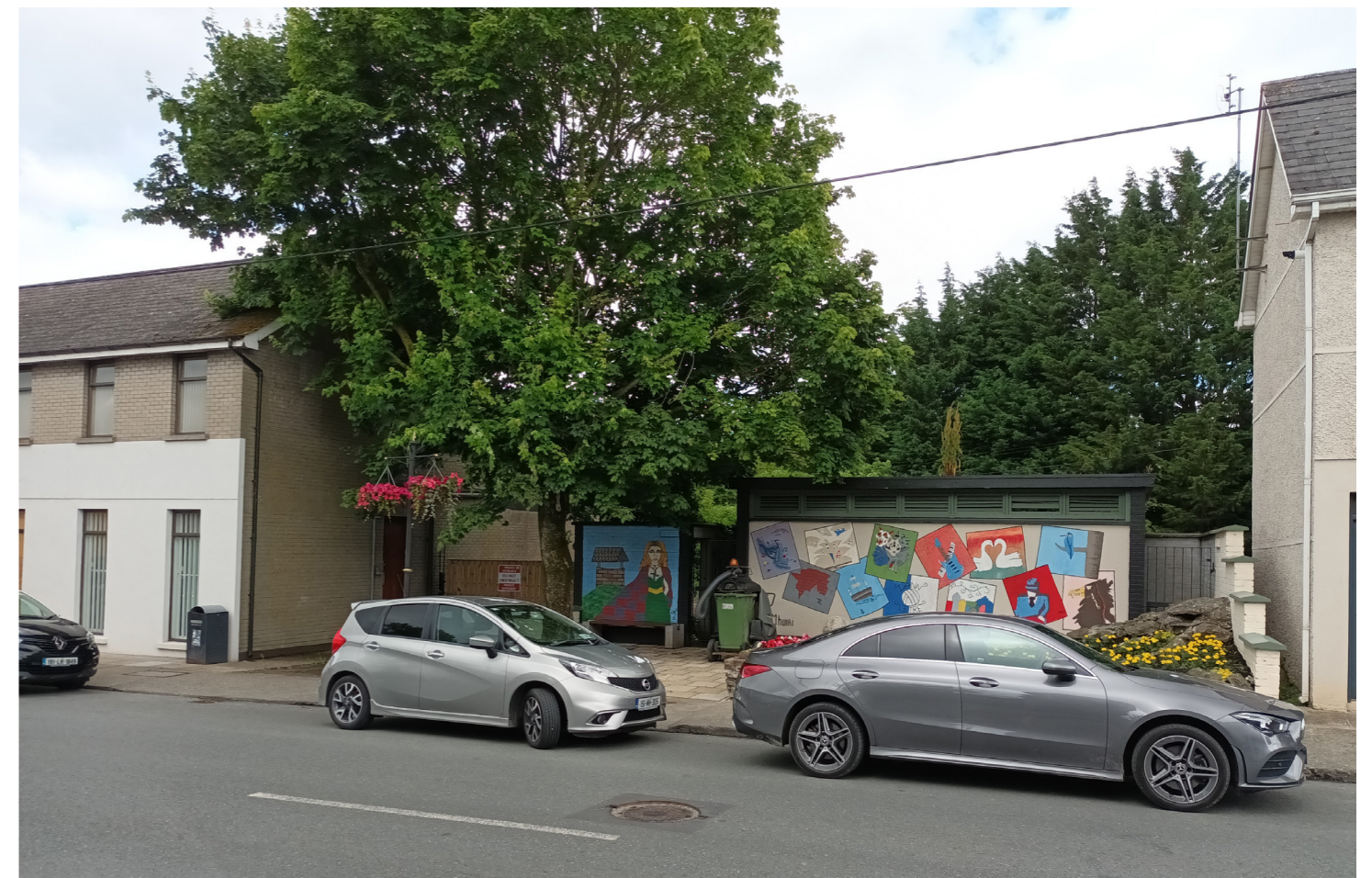
Fig.133 - View of the existing Library and public toilet block from the Main Street
