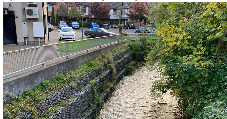
Fig.104 - Treatment of river embankment in the Forge
