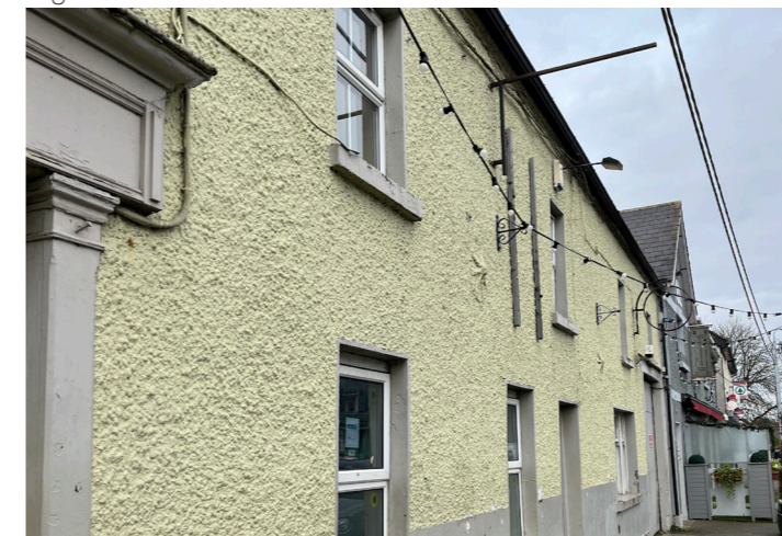
Fig.162 - Existing facade condition of the Corner House Pub
