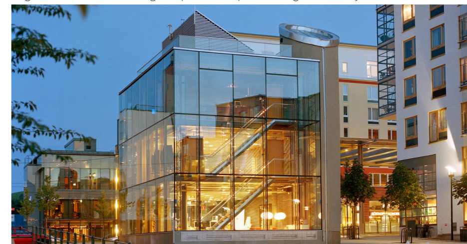
Fig.158 - GlashusEtt energy centre, Stockholm, Sweden.
