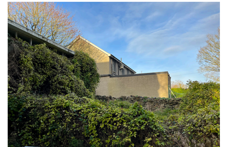
Fig.120 - Rear of former Bol building showcasing level change
