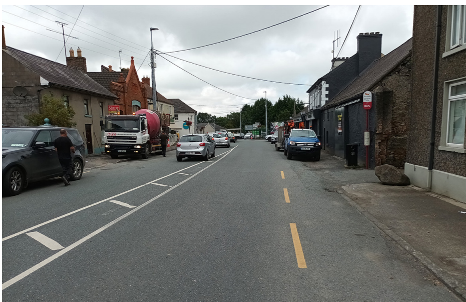
Fig.25 - Image of bus stop in Upper Main Street, highlighting the lack of seating or shelter, and the excessively narrow footway. The lack of lay-by means the bus blocks the road when stopped.
