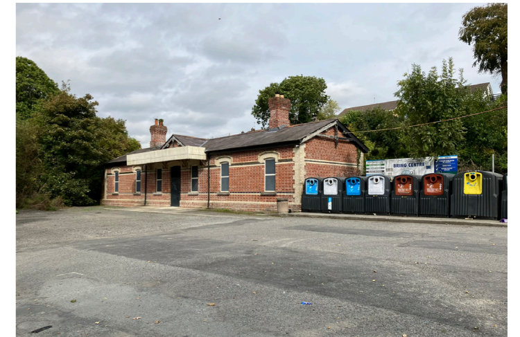
Fig.139 - View of existing train station
