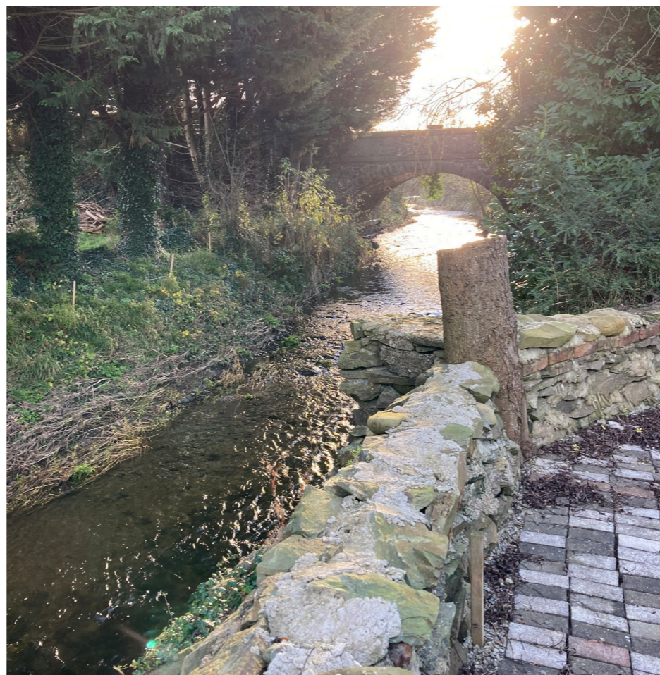
Fig.77 - White River - view of Station Road bridge
