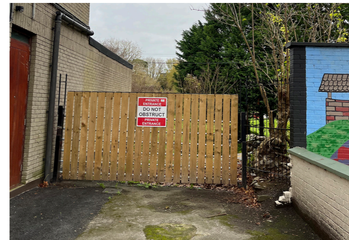
Fig.118 - Fenced access to private right of way
