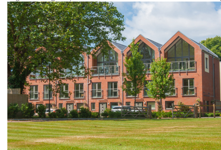
Fig.61 - Graylingwell housing, Chichester, UK - JTP Architects
