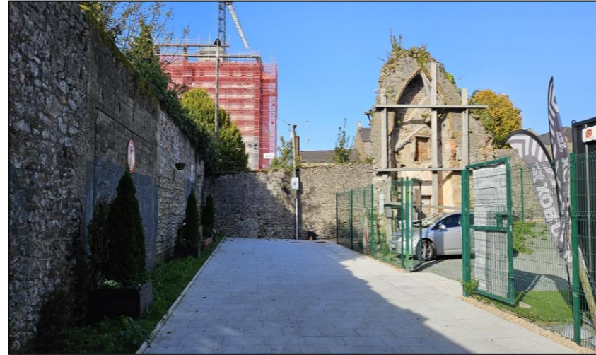
Photo 13: West Gable of the North Aisle
