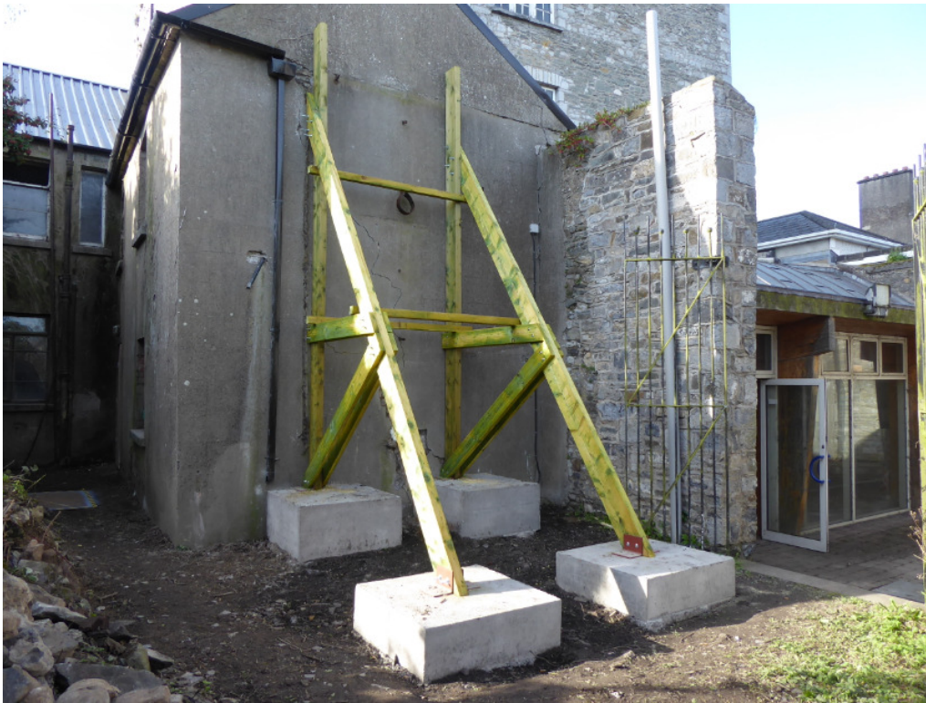
Fig 2.9 – Remedial buttress to the Judges' Chambers
