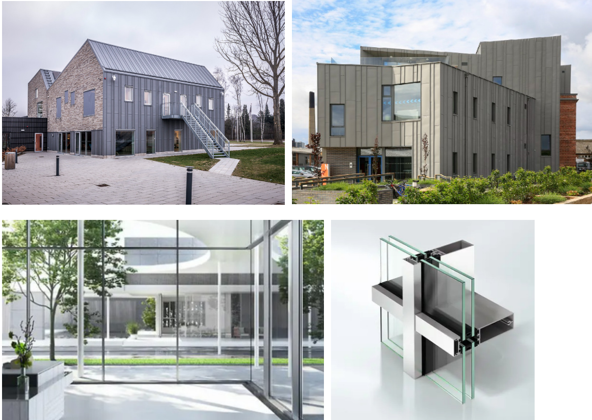
Fig 5.4 – Standing-seam zinc cladding and aluminium-framed curtain walling
