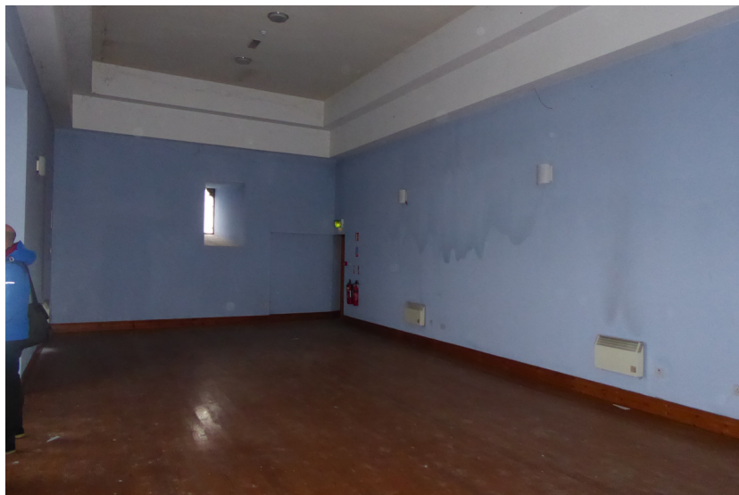
Fig 5.17 – Dry-lining of Grand Jury Room – to be removed.
