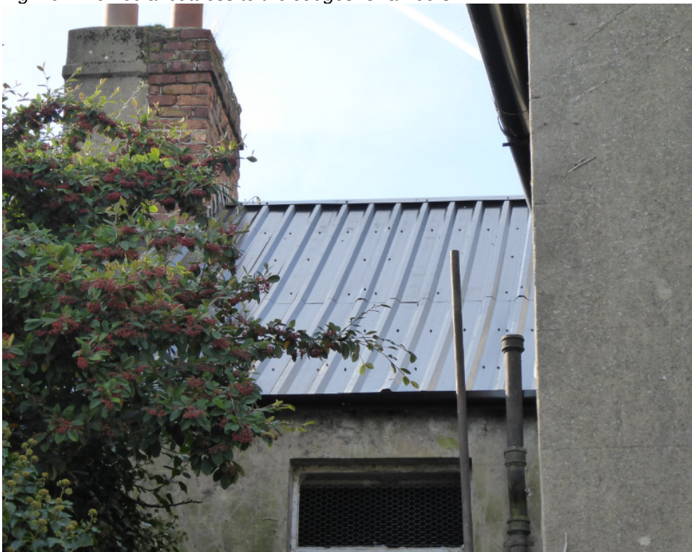
Fig 2.10 – Replacement roofing to the Judges' Chambers
