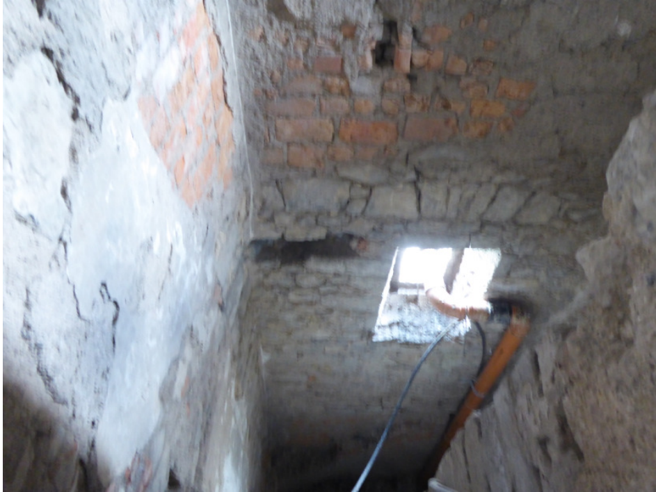
Fig 5.15 – View into the (blocked up) garderobe
