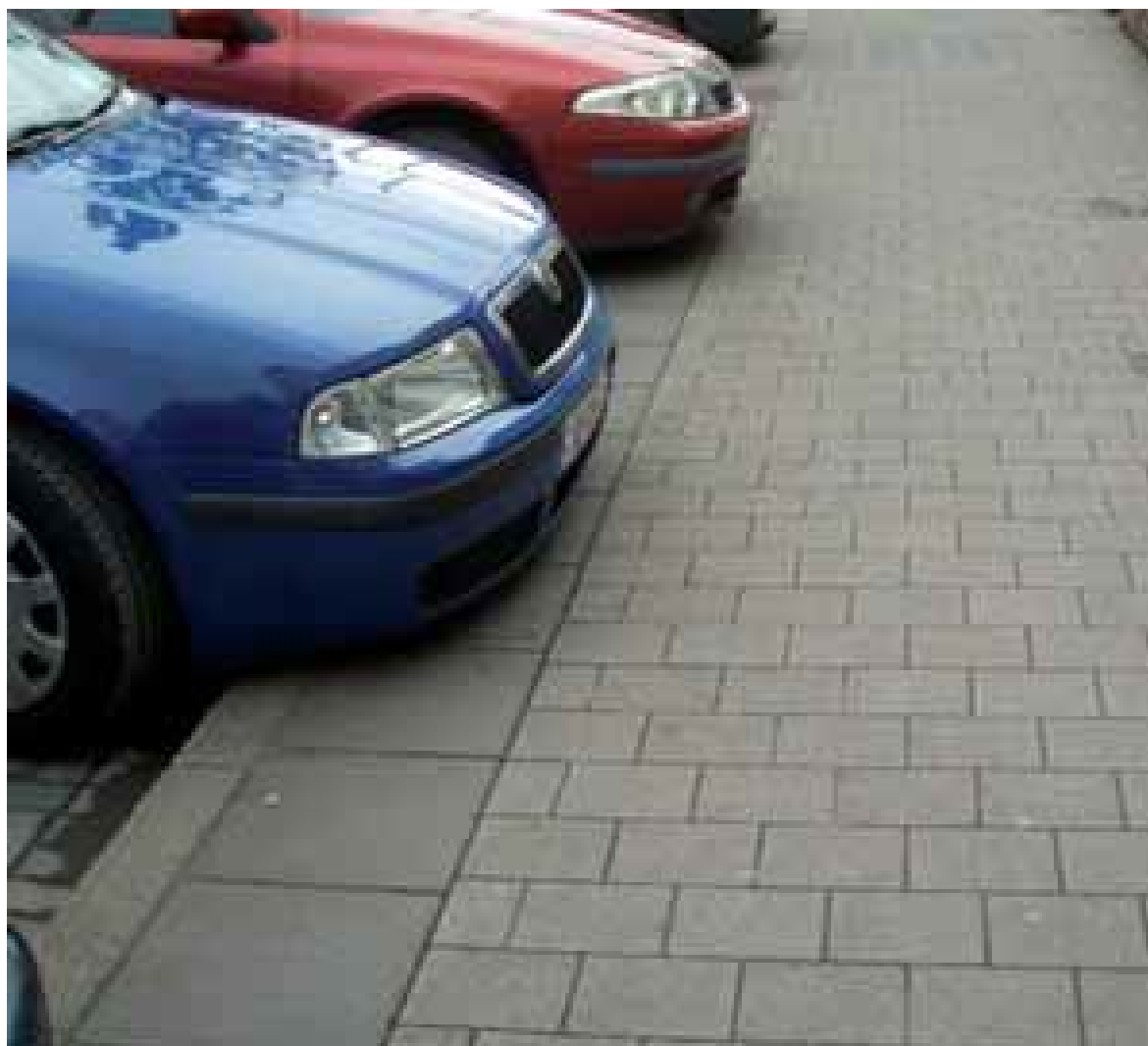
Figure 4.36: An example where a narrow verge is provided to ensure that vehicle overhangs do not intrude on the footway (DMURS)
