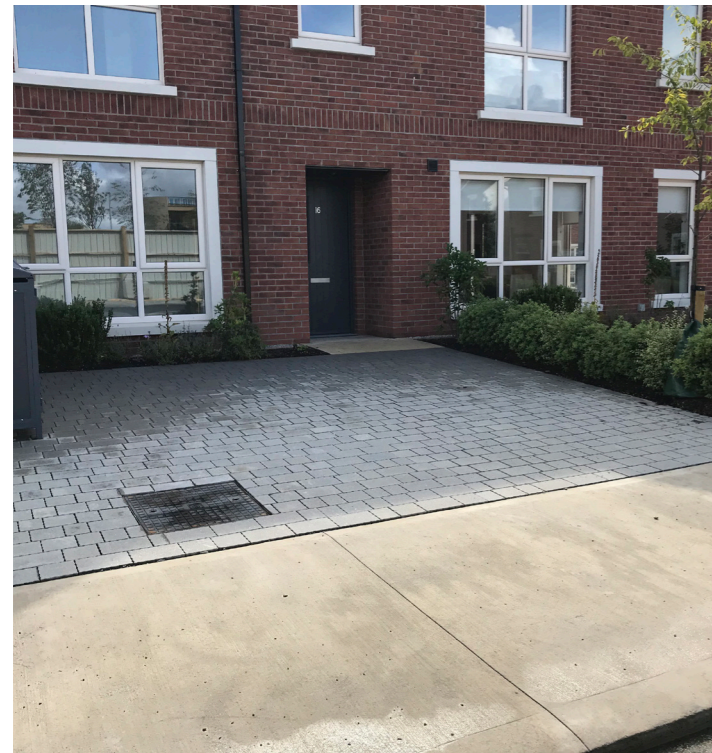
Brushed concrete public footpaths
