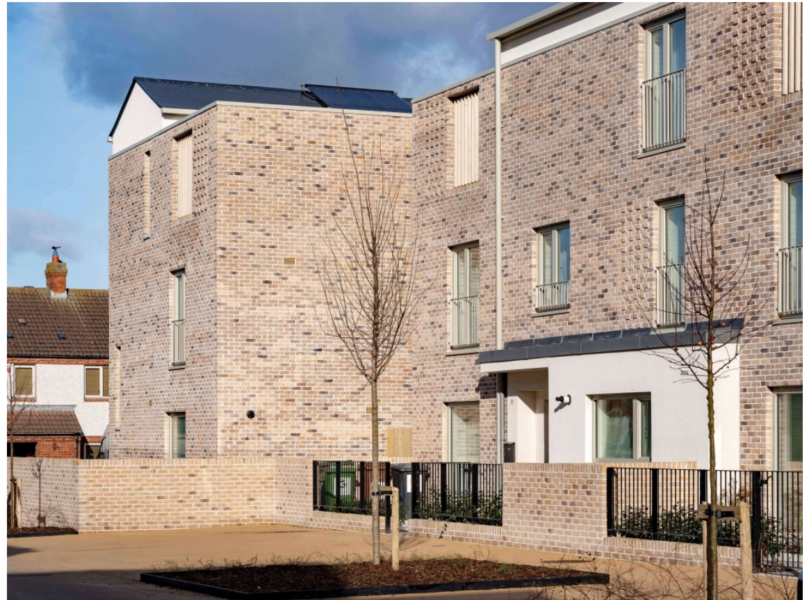
CLOCKWISE FROM TOP: EXAMPLE OF BUFF BRICK MIX PAIRED WITH METAL PROJECTING DETAILS AND AREAS OF RENDER (ROSEMOUNT COURT, DÚN LAOGHAIRE-RATHDOWN COUNTY COUNCIL); BUFF BRICK SAMPLE; TYPICAL OFF-WHITE ACCENT RENDER.
