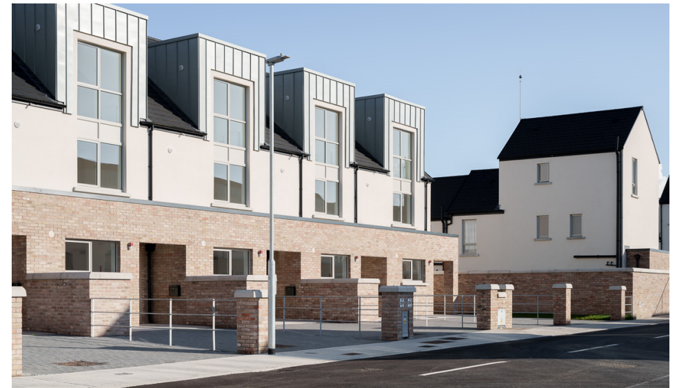
BELOW RIGHT: PHOTOS OF CHURCHFIELDS SOCIAL HOUSING BY EML ARCHITECTS FOR FINGAL COUNTY COUNCIL, SHOWING PERMEABLE PAVING USED FOR OFF-STREET PARKING.
