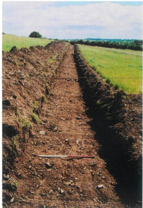
Plate 4: Trench 6, Field 2, from east (CP1:16)
