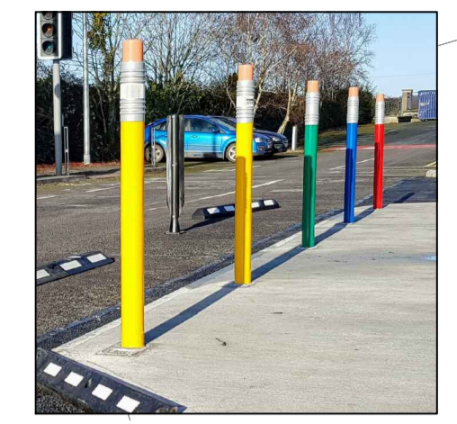
YELLOW/GREEN/RED PENCIL BOLLARDS AT SCHOOL ZONE PLACED ON TOP OF EXISTING KERB
