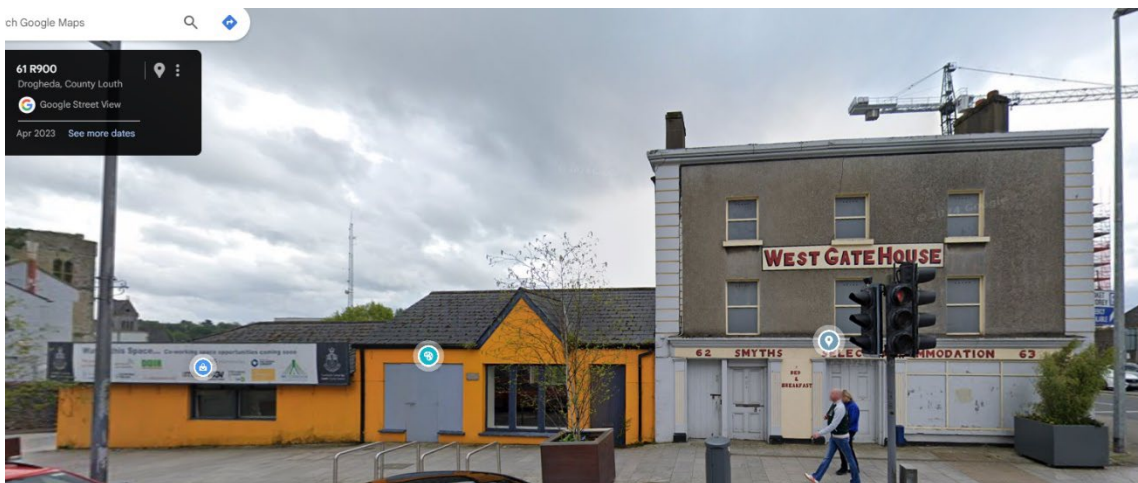
Figure 1: Westgate House, Drogheda
