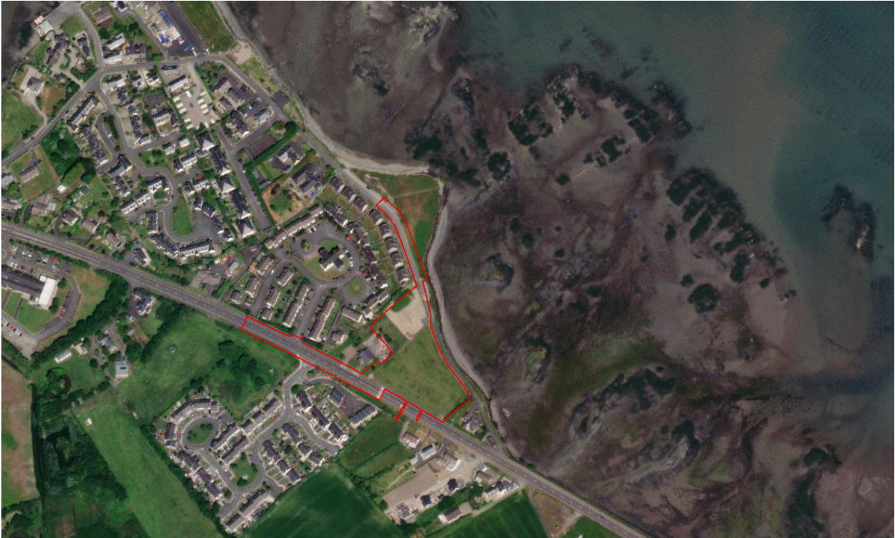
Figure 2-3: Extent of Proposed Development - Car Park and Tennis Court Area shown bound in Red
