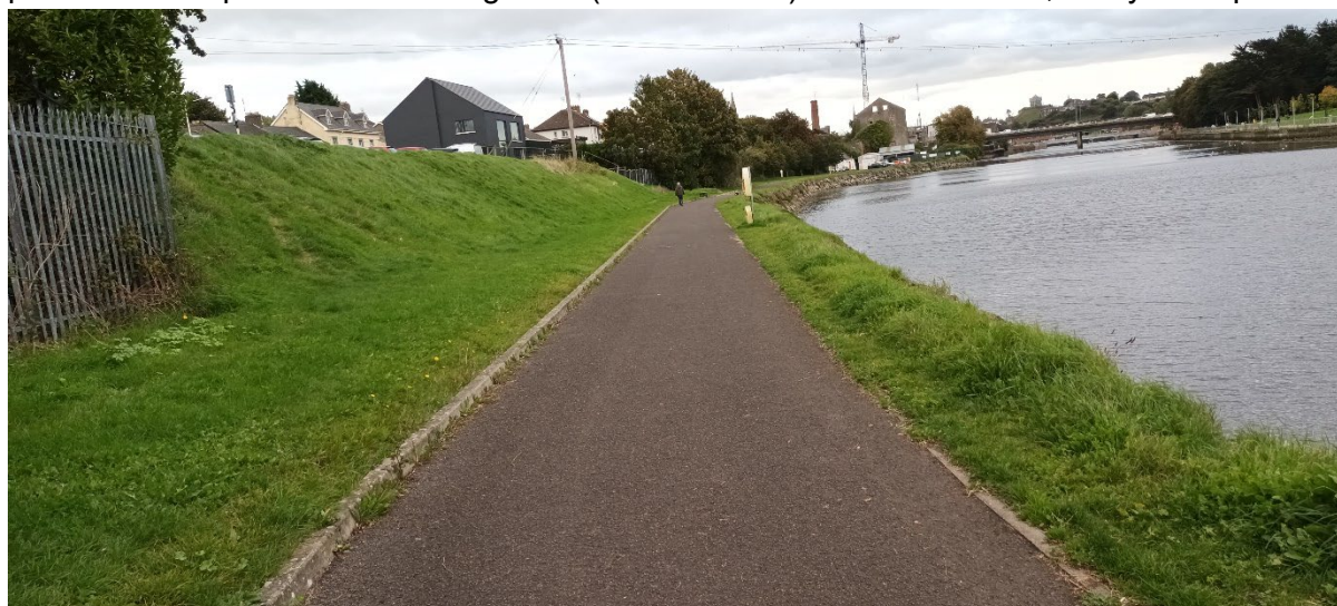
Plate 1.1. Existing Pathway within SAC boundary
