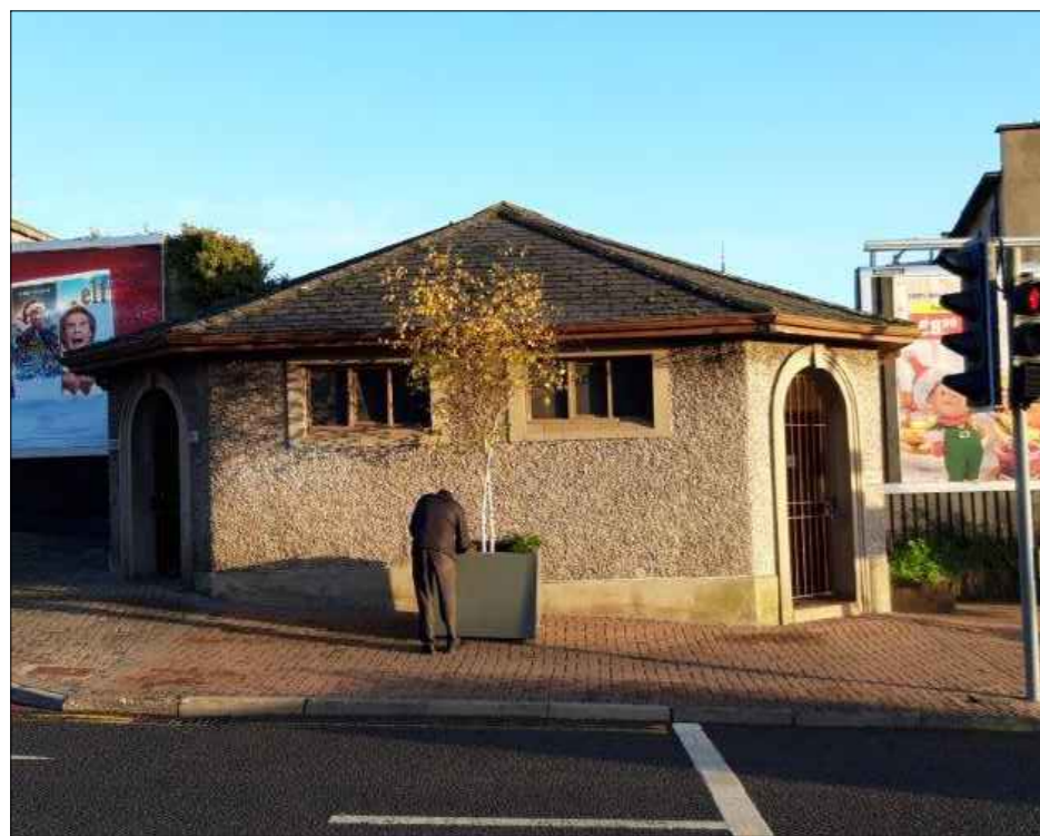
Photo of the Existing Toilet Block's Northern Elevation
