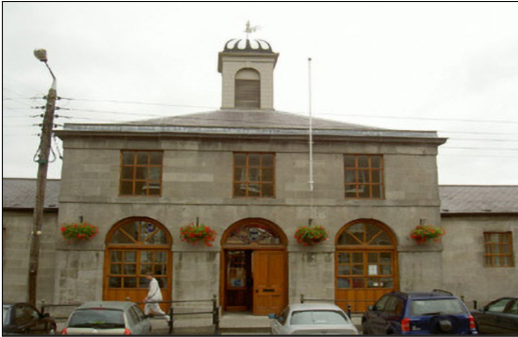
Photo 27: General view showing the late C18th former Cornmarket, on the north side of Fair Street, close to the north-east corner of the Westgate Project Area. The Cornmarket was designed by noted Irish Architect Francis Johnston and has national significance. It has been converted to use as the Local Authority offices over a century ago.
