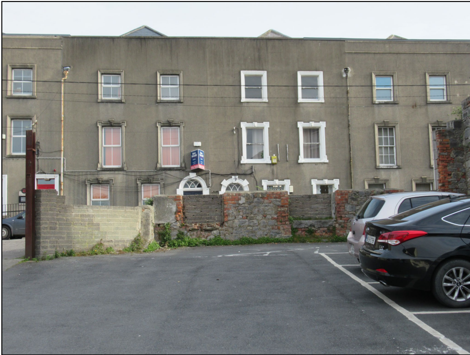
Photo 22: General view looking north, showing the fine terrace of houses standing on the north side of Fair Street. The formerly gabled roofs can be seen above the flat front parapets.
