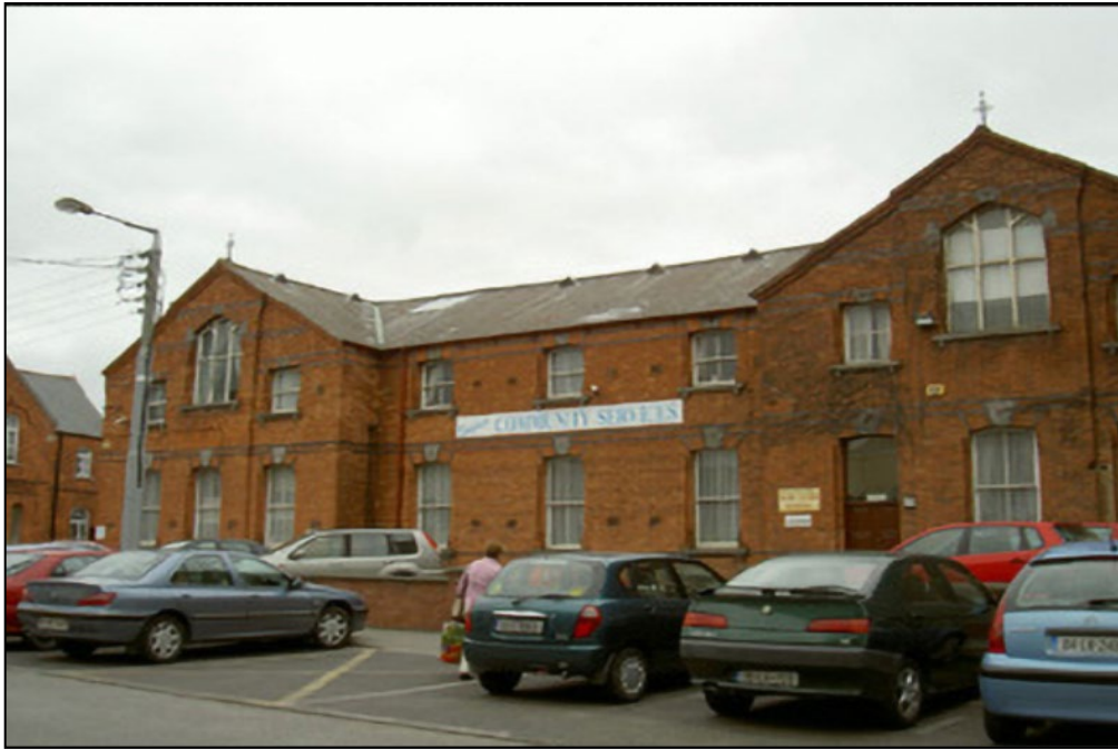
Photo 29: General view showing the school attached to the former Convent of the Sisters of Charity, on the north side of Fair Street. This structure is currently being redeveloped as part of the Local Authority Offices.
