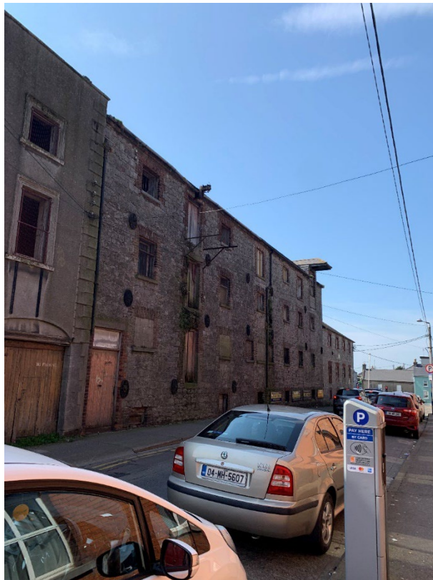
Plate 16.8: Industrial warehouse on Fair Street, facing southwest
