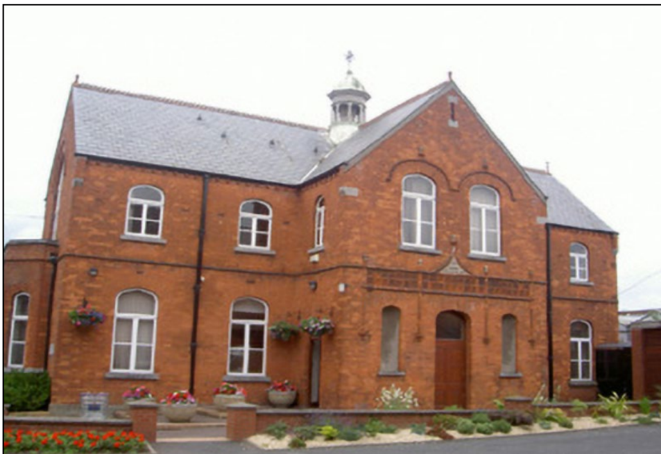
Photo 28: General view showing the former Convent of the Sisters of Charity, on the north side of Fair Street, adjacent to the former Cornmarket. This structure is currently being redeveloped as part of the Local Authority offices.
