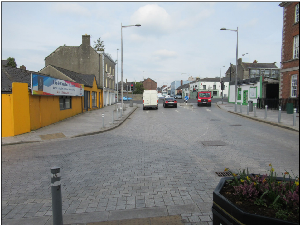
Photo 11: General view showing west along West Street, towards the location of the long demolished Westgate. Barlow House is at the right edge of this photo. West Gate House is the three-storey structure left of centre.
