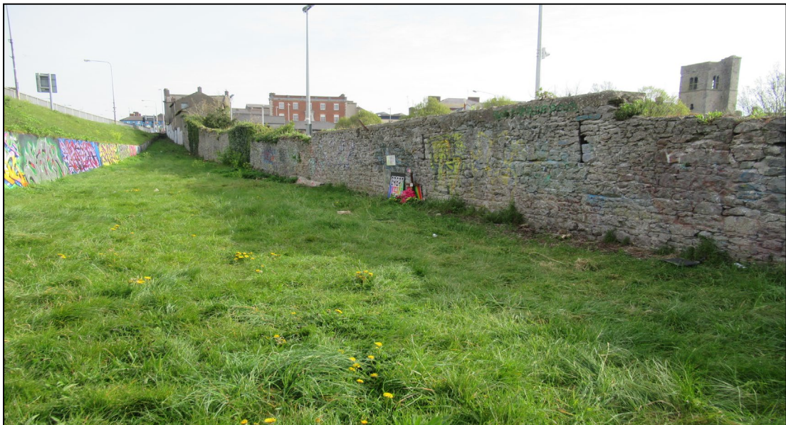
Photo 1: General view looking north, showing the extent of the surviving town walls, running from the river Boyne up to the since demolished West Gate.
