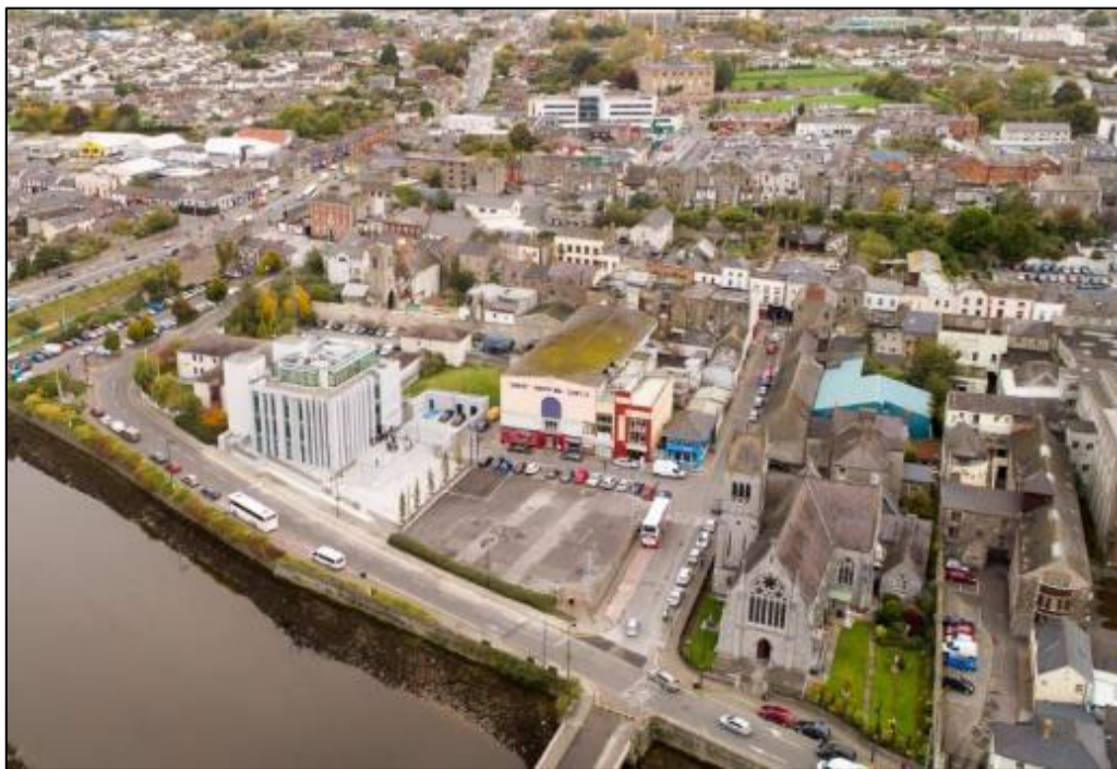
Photo 18.4 Aerial Image of the Application Site and Immediate Surroundings (Source: www.westgatevision.ie )
