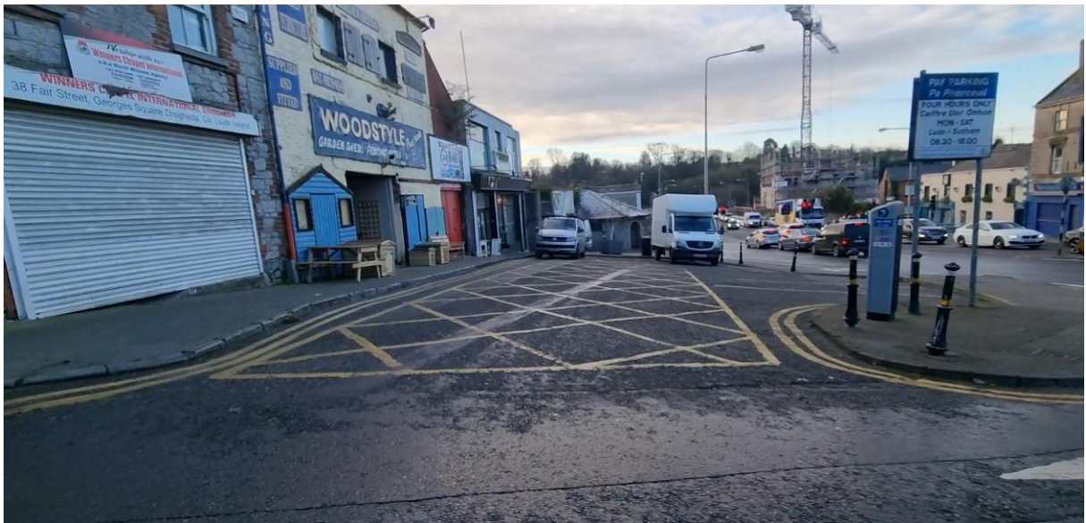
Figure 11: Existing Parking to be removed at location of proposed corten plate, walkway and stepping terraces, south of Fair Street
