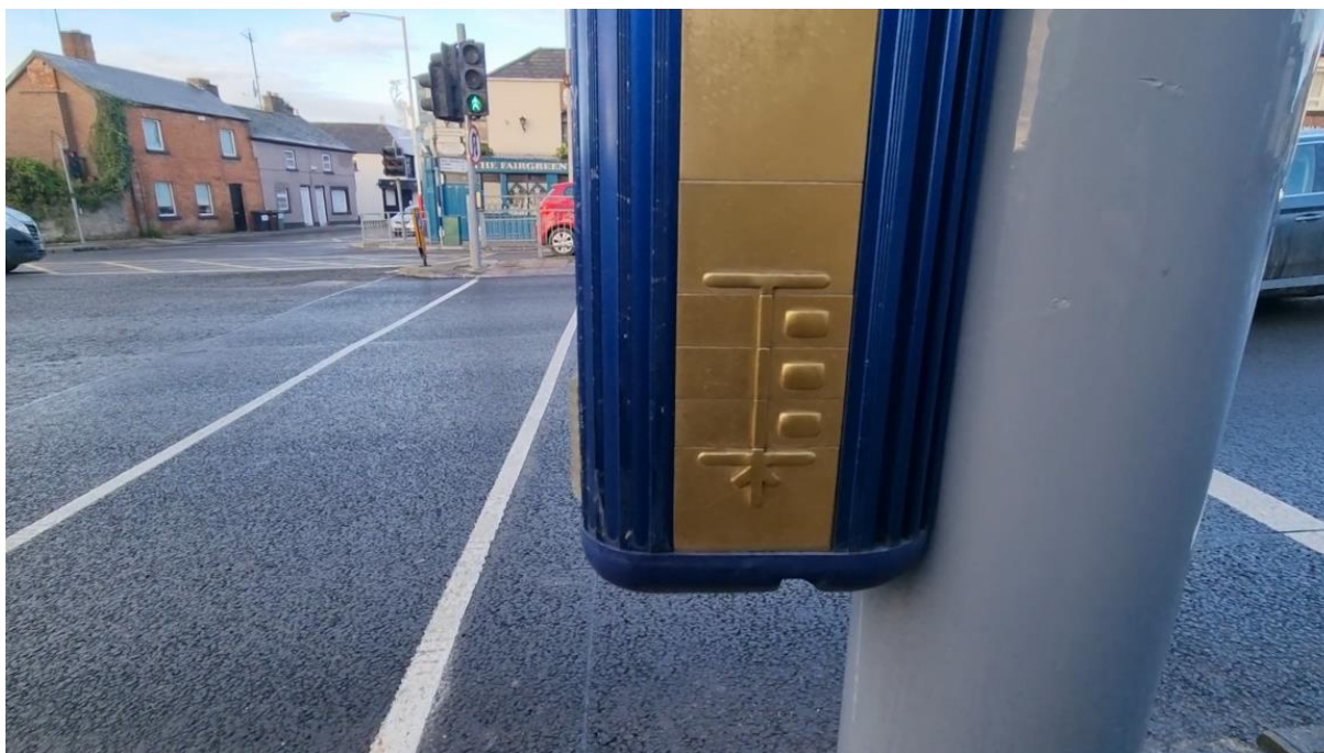
Figure 48: Existing Tactile Mapping on northeastern side of signalised crossroads
