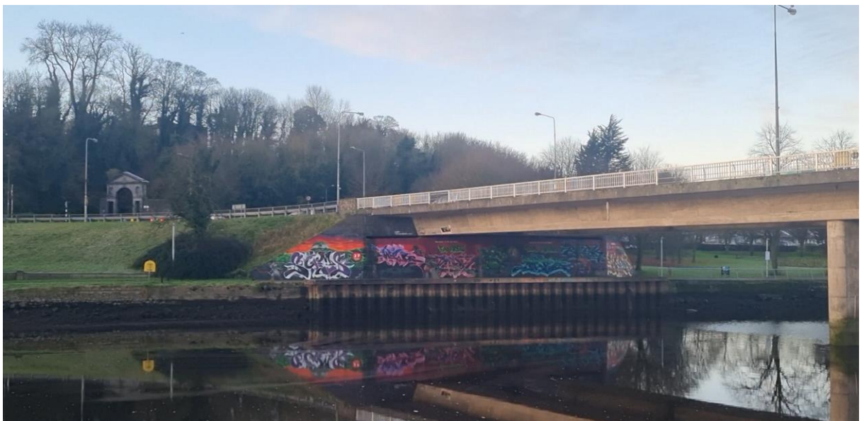
Figure 67: Cycling Route to continue Underneath Peace Bridge
