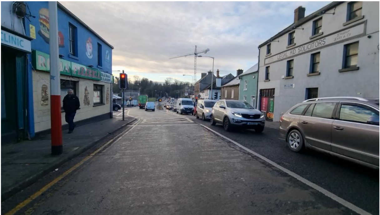
Figure 24: Existing Anti-skid surfacing on approach to existing traffic signals
