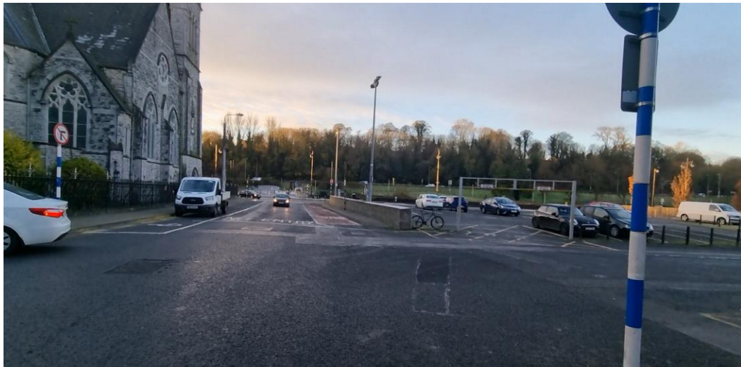
Figure 136: No provision for no right turn signs out of new car park access/egress on Dominic St
