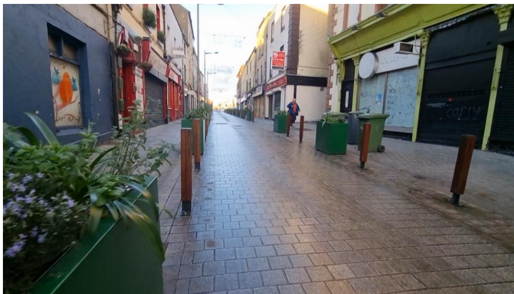
Figure 145: No Clearance to Existing Street Furniture on West Street
