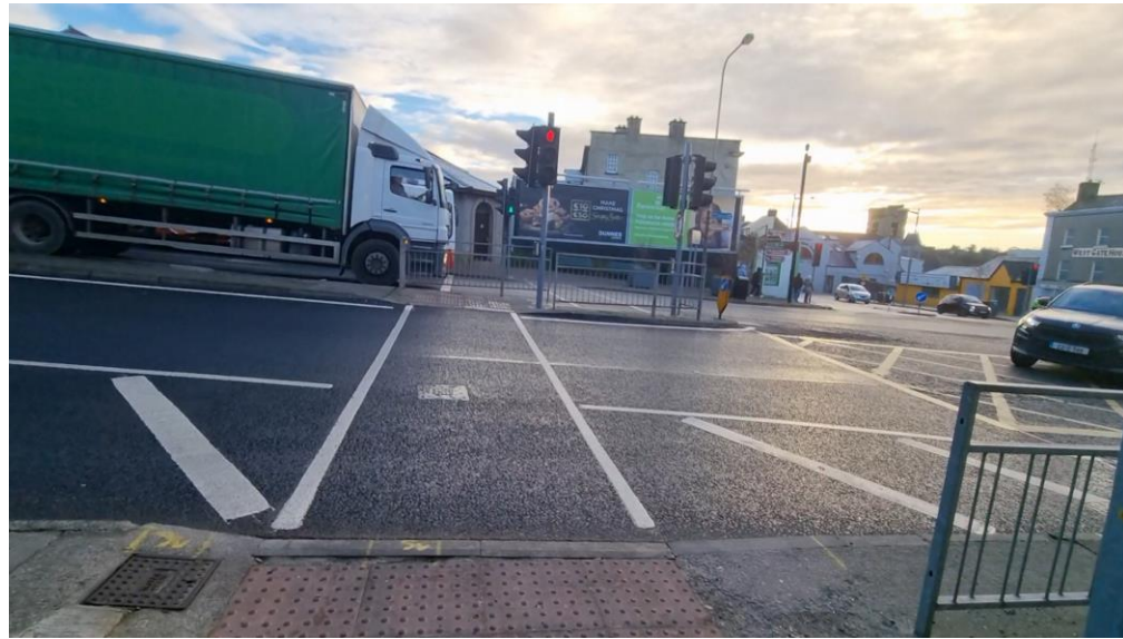
Figure 104: Existing Sheep Pen Arrangement and narrow crossing
