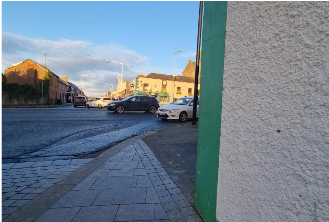
Figure 84: Limited intervisibility to/from right at Crossing on Trinity Street
