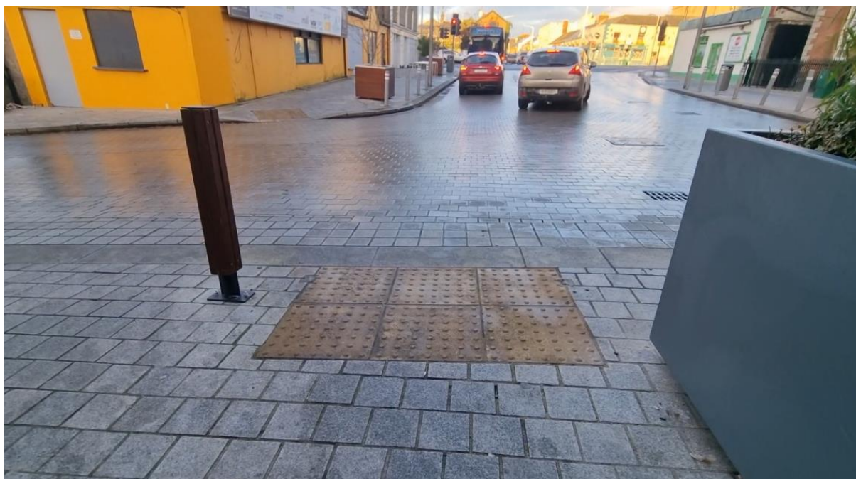
Figure 82: Existing informal crossing point across mount of junction with Father Connolly Way/West Street to be removed. Note Tactile is incorrectly aligned at present
