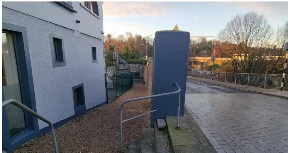
Figure 86: View southwards showing level differences at retaining wall
