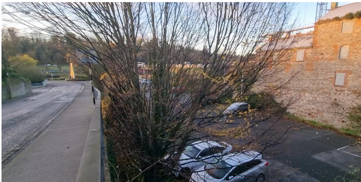
Figure 103: Significant level difference between Car Park and Father Connolly Way
