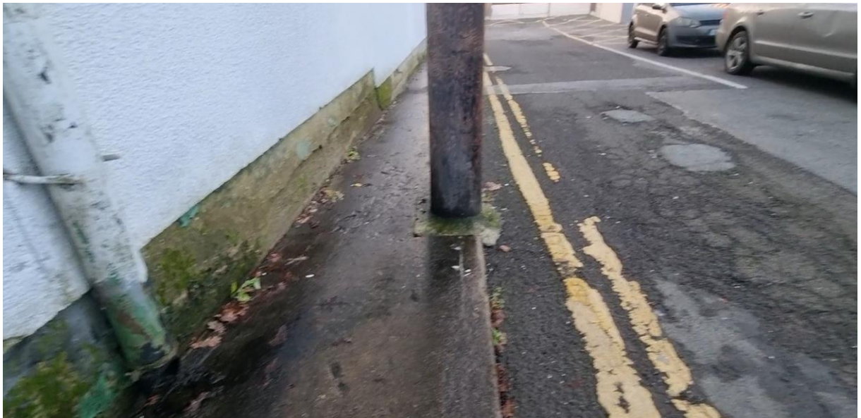
Figure 7: Utility Poles obstructing narrow Footways with no clearance to carriageways
