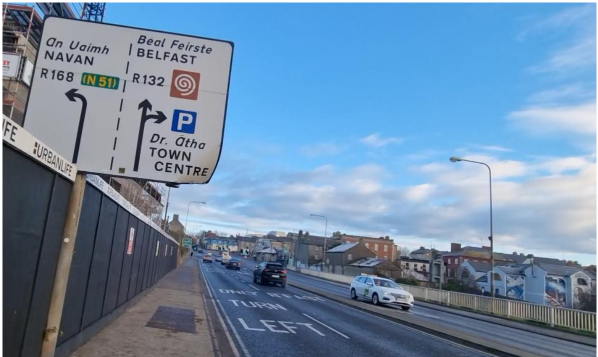
Figure 121: Existing Map Sign to be Replaced to reflect new layout Note: Sign too close to carriageway edge has been struck
