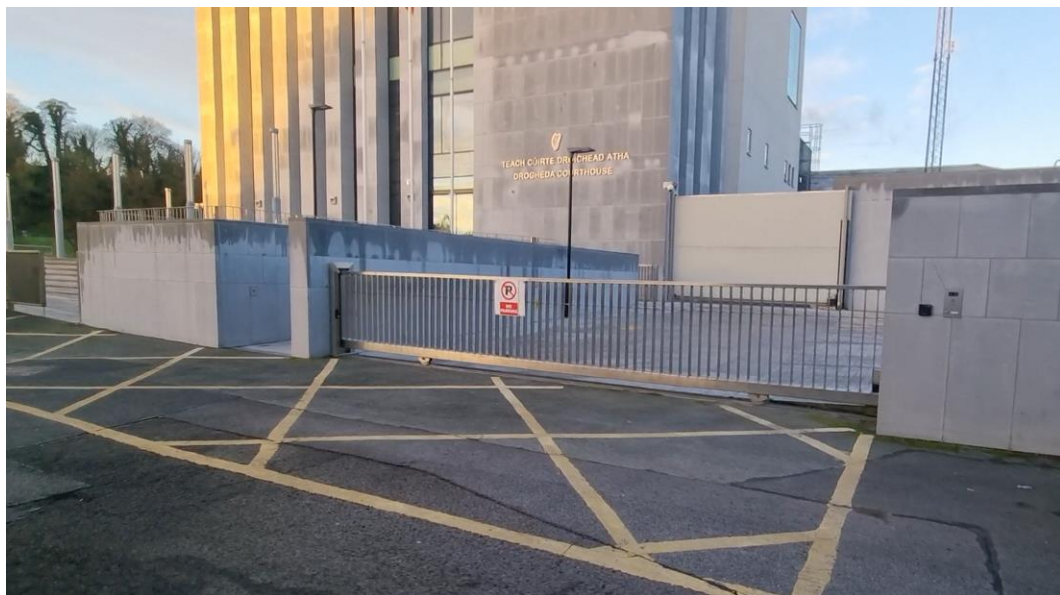
Figure 144: Design Plans do not show provision for yellow box markings Or vehicular access at Courthouse
