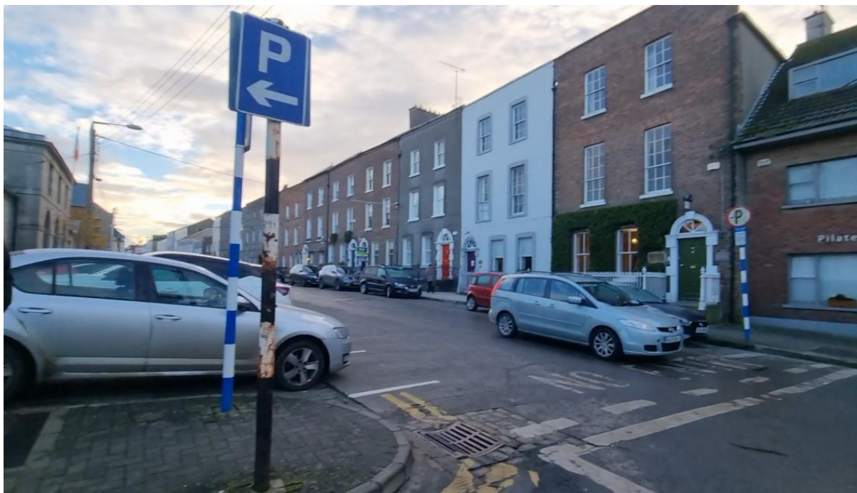
Figure 61: Existing Visibility to the right from junction opposite Scholes Lane currently obstructed by vehicles parked within perpendicular parking bays adjacent
