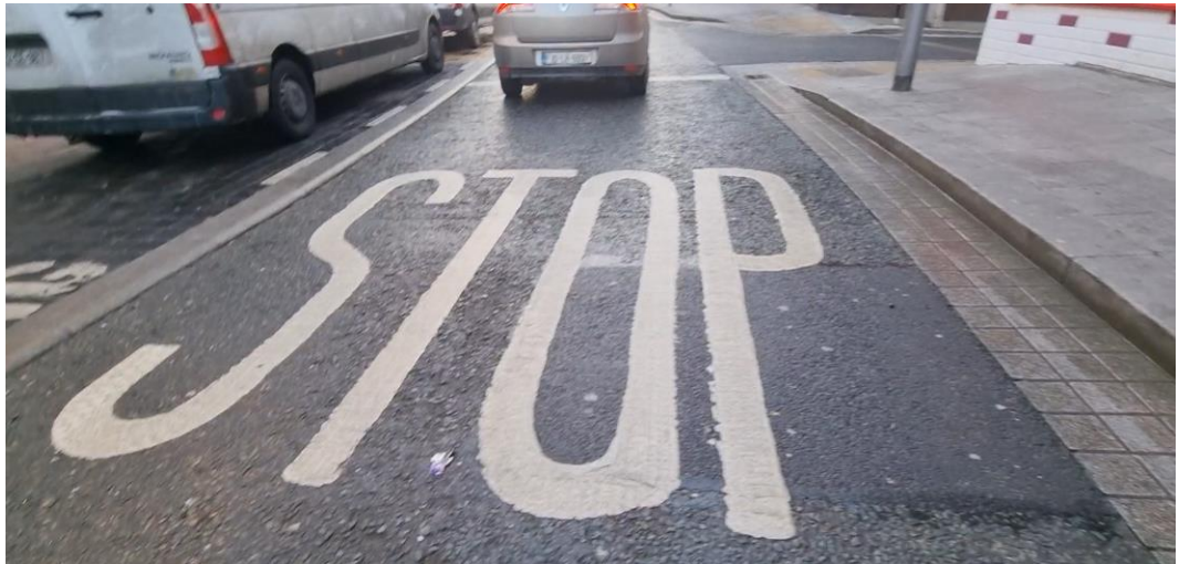
Figure 141: Existing Stop Markings removed on western arm of intersection of Dominic street/ West Street
