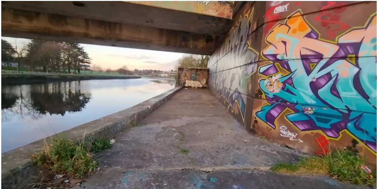
Figure 66: Cycling Route to continue Underneath Peace Bridge
