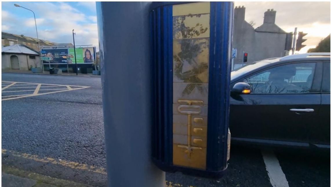
Figure 47: Existing Tactile Mapping on southwestern side of signalised crossroads
