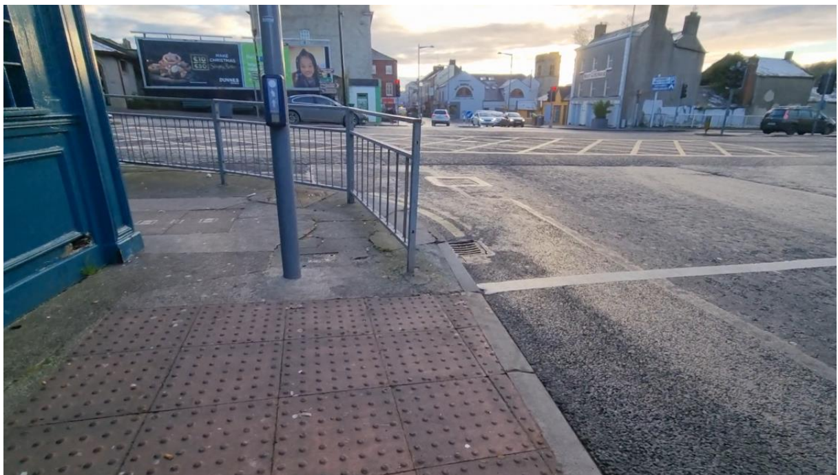
Figure 45: Signal head poles obstructing footway on Trinity Street
