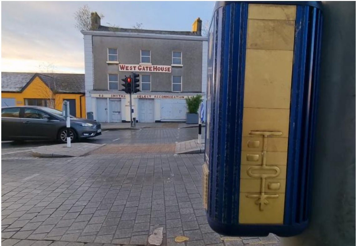
Figure 46: Existing Tactile Mapping on Eastern side of signalised crossroads
