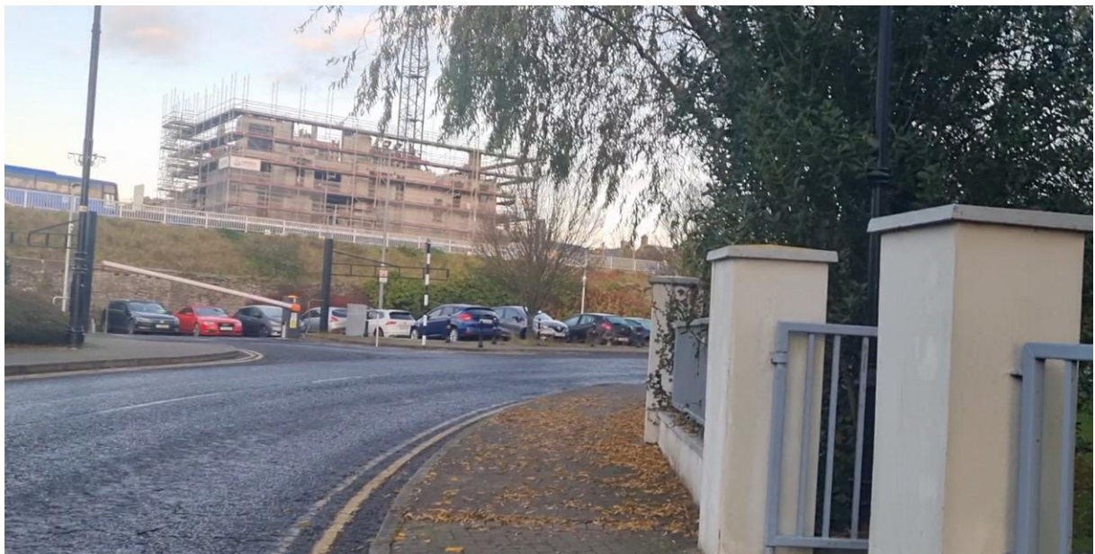
Figure 39: Boundary Treatment reducing intervisibility for pedestrians wishing to cross on desire line to/from car park on Father Connolly Way
