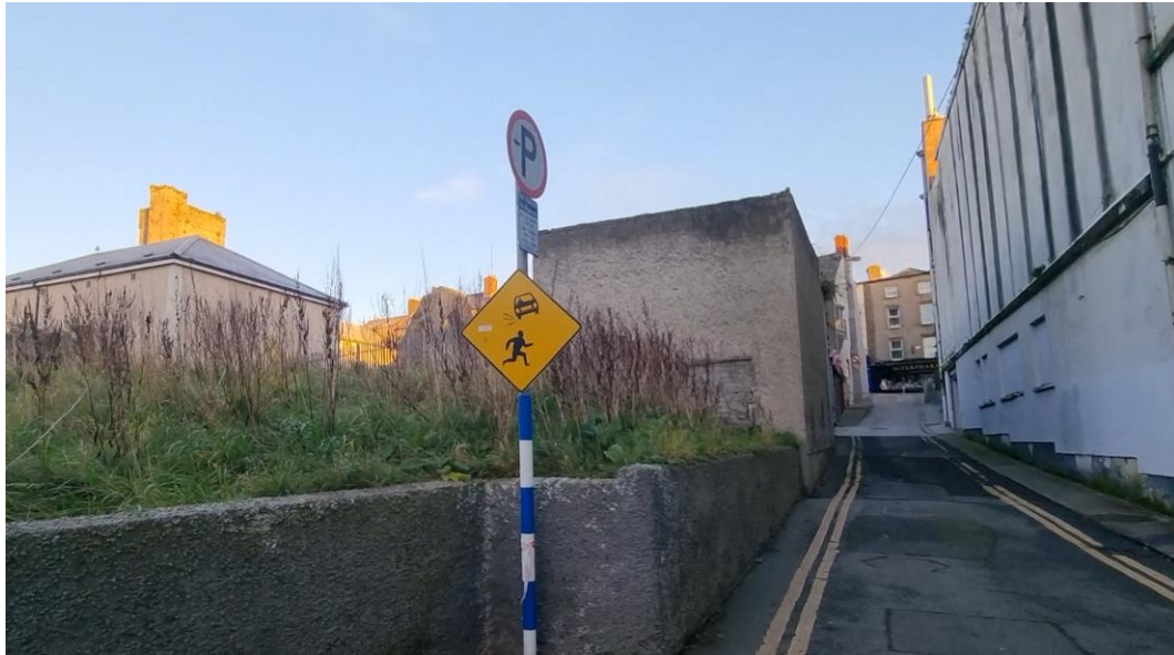
Figure 143: Existing Pedestrian Warning Signs used where intervisibility is poor
