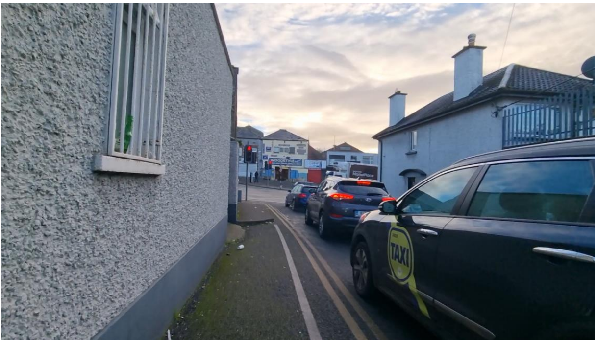
Figure 99: Footway terminates abruptly at scheme ti-in on Fair Green
