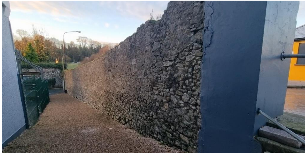
Figure 87: Eastern side of retaining wall on Old Abbey Lane
