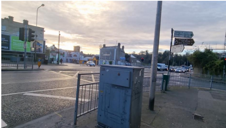
Figure 106: Visibility to right compromised by utility cabinet location
