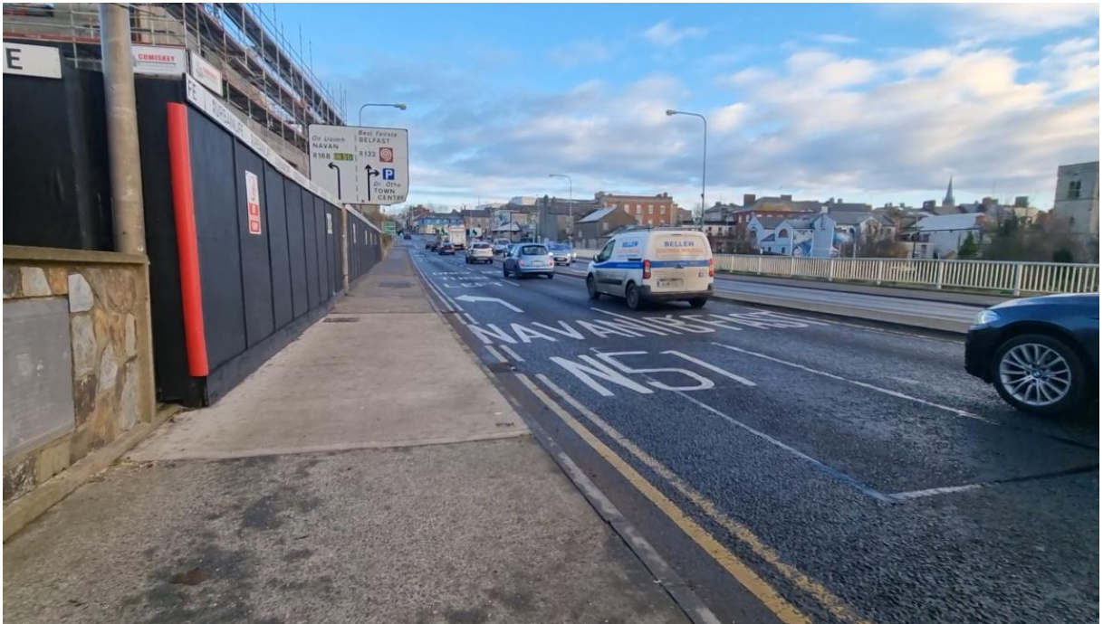
Figure 120: Old Road Markings to be Removed
