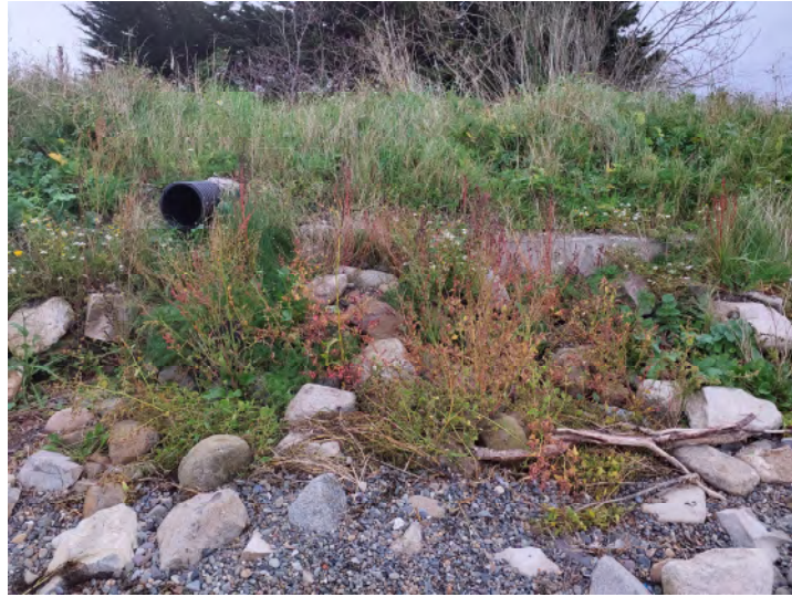
Plate 17. Ground photograph taken on the 7 th October, 2023 at Chainage 212m facing in a northerly direction towards Location B Coastal Works Area showing land drainage pipe
