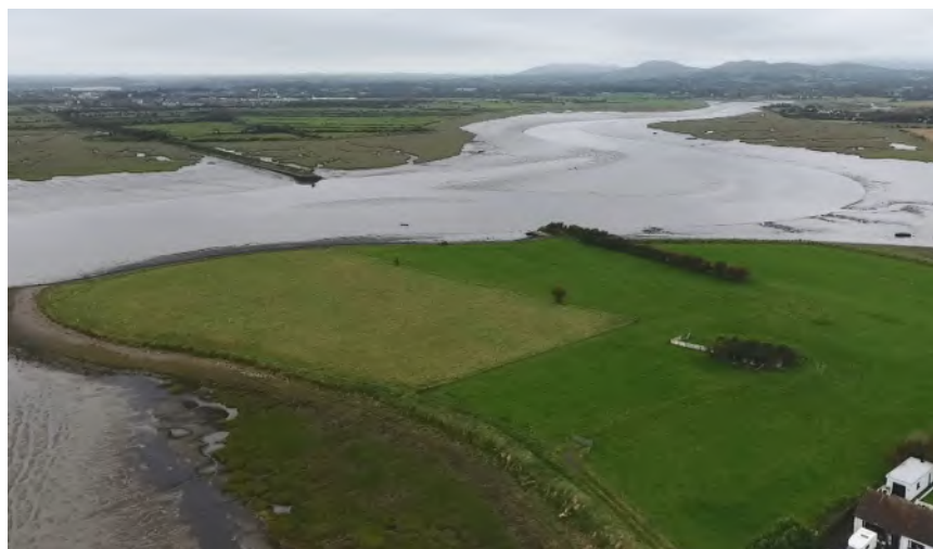
Plate 13. Aerial photograph taken at 70m elevation at Bellurgan Quay facing in a north-westerly direction showing the abutments for the former Dundalk to Greenore Railway Bridge
