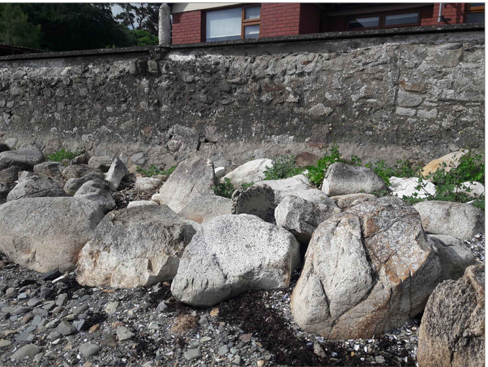
Image P4 View of existing rock armour (non effective)
