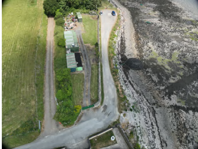
Plate 8. Aerial photograph taken over the adjacent residence at 40m elevation facing in a northerly direction showing the commercial enterprise to the north of the site.
