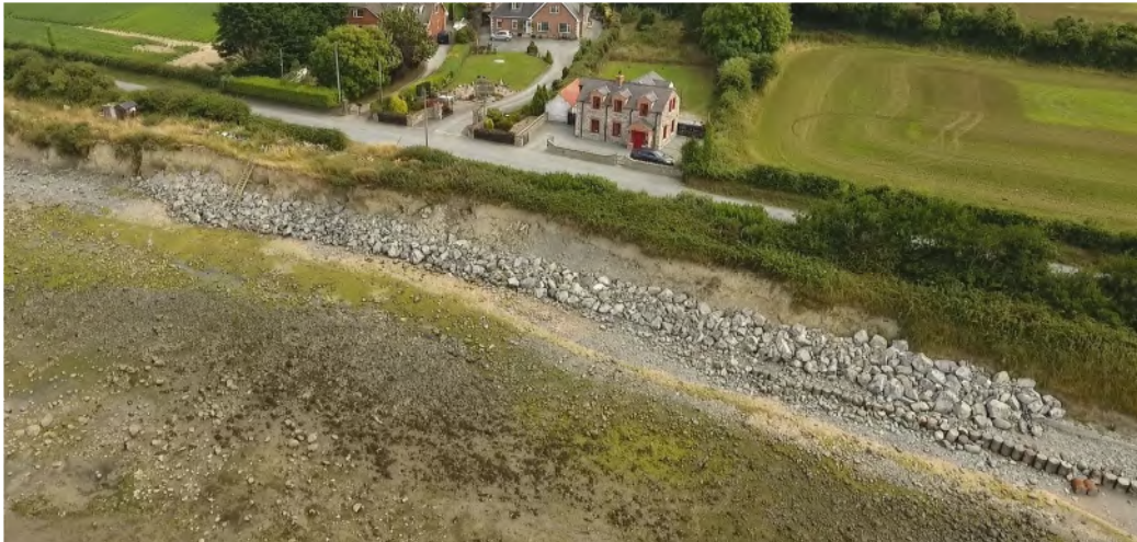
Plate 2. Aerial photograph of rock armour constructed to prevent coastal erosion at Salterstown, Annagassan, County Louth.
