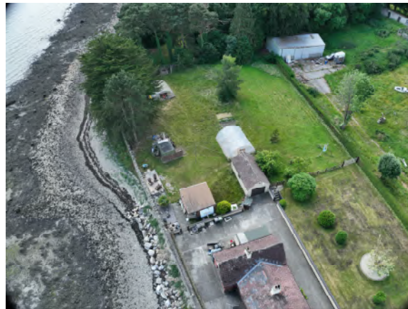
Plate 7. Aerial photograph taken over the works site at 40m elevation facing in a southerly direction showing the property to the south of the site and adjacent mixed broadleaf/conifer woodland which is the northern boundary of Omra Park
