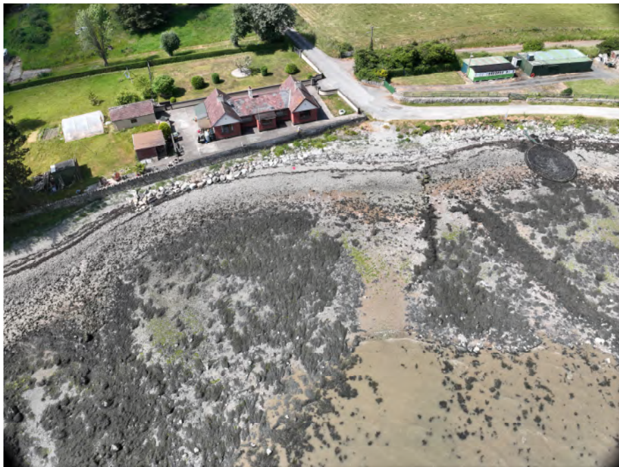
Plate 1. 4K Aerial photograph taken at an elevation of 40m above ground level approximately 100m to the east of the site facing in a westerly direction towards the location for the proposed coastal protection works located to the east of the residence
