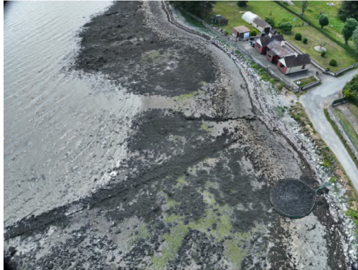
Plate 9. Aerial photograph taken at a location to the northeast of the works site 40m elevation facing in a southerly direction showing the pipe running along the foreshore
