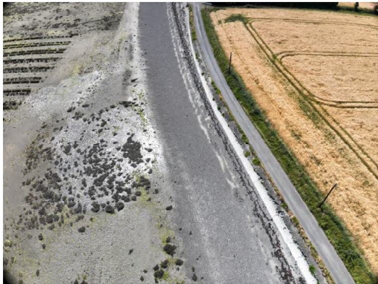
Plate 2. 4K Aerial photograph taken at 40m elevation over foreshore facing in a southerly direction showing the northern end of the damaged seawall with collapsed concrete capping
