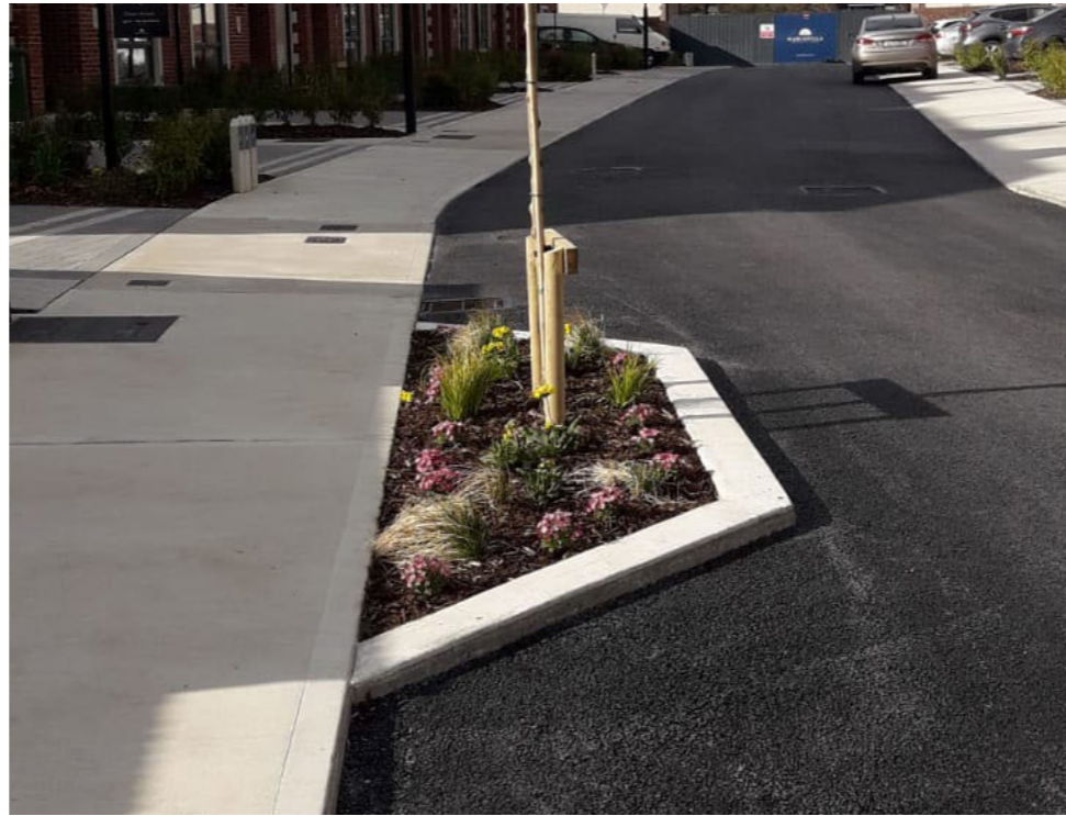
Street trees - build-outs used to define parking areas and to provide horizontal deflections for traffic calming
