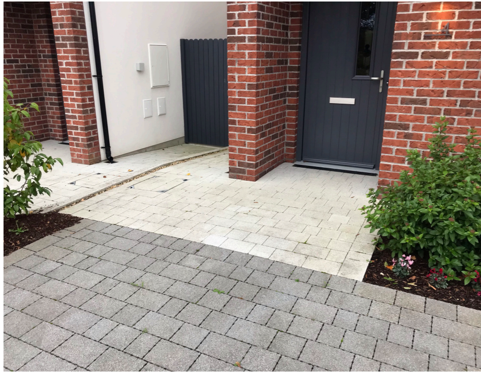
Precast concrete paving blocks in graphite and light grey colours. Graphite used exclusively beneath parking areas to limit visible staining. Lighter colours used to highlight dwelling entrances and approaches. Driveways to use permeable paving generally.
