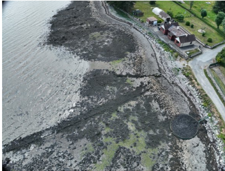
Plate 9. Aerial photograph taken at a location to the northeast of the works site 40m elevation facing in a southerly direction showing the pipe running along the foreshore
