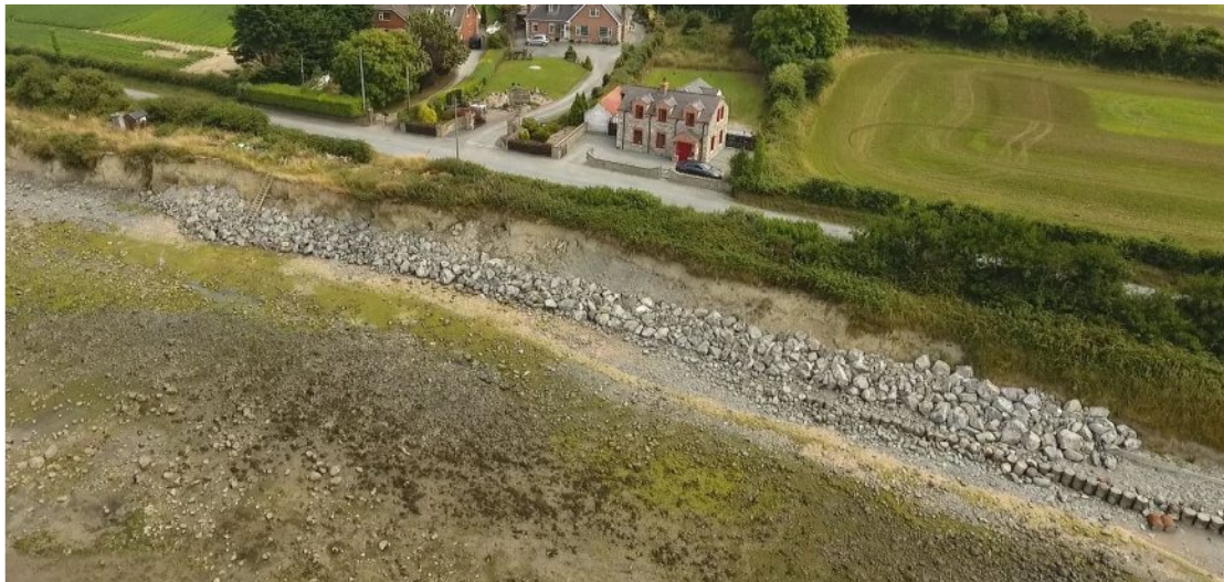
Plate 2. Aerial photograph of rock armour constructed to prevent coastal erosion at Salterstown, Annagassan, County Louth.
