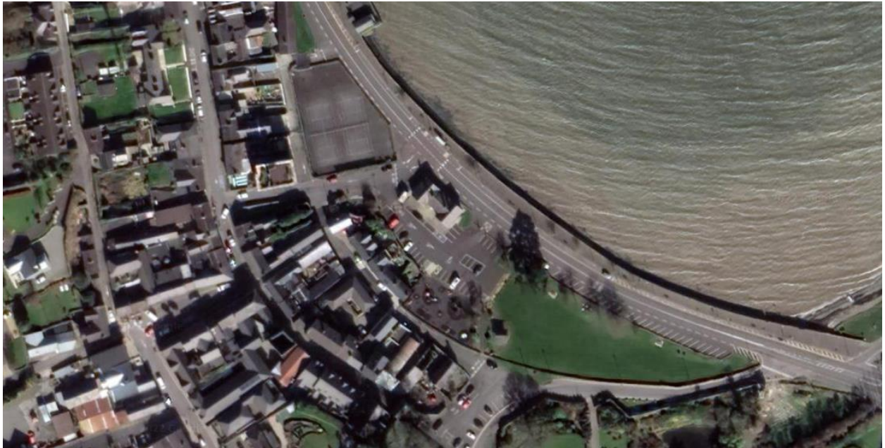
Aerial View of Carlingford Town Centre
