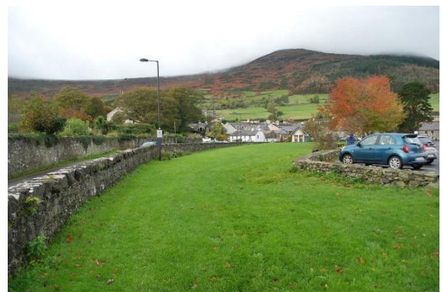
Wall of C18 th Quay (LHS) Infilled for railway
