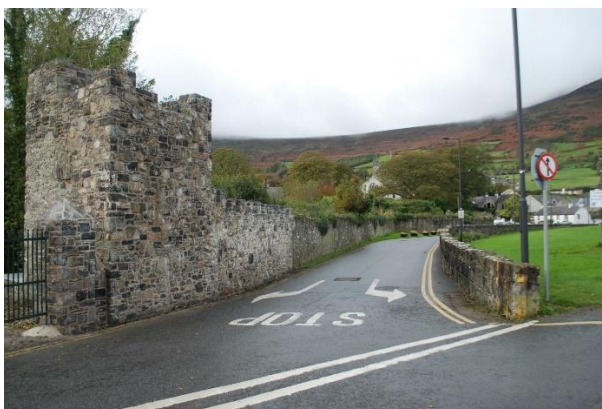
1800's Historic Former Quay Wall to RHS
