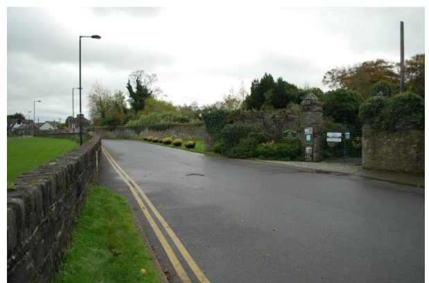
1800's Former Quay Wall bounding to road to LHS
