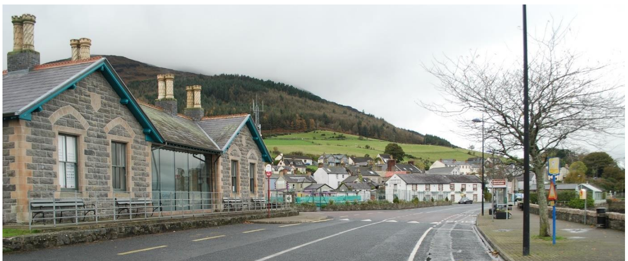
Greenore Road dominates the frontage and the setting of the Tourist Office with little dwell space
