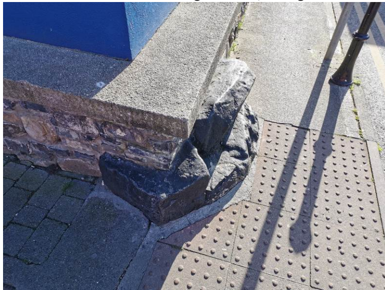
Plate 23 View of CH16, facing southeast
