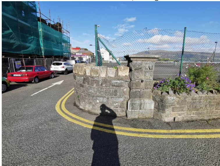
Plate 39 View of stone pier and stone wall To CH28, facing north
