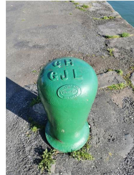
Plate 46 View of cast-iron mooring posts to CH32, facing northeast
