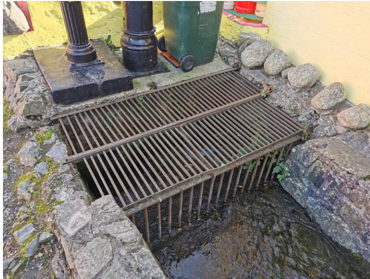
Plate 29 View of grate to CH20, facing east
