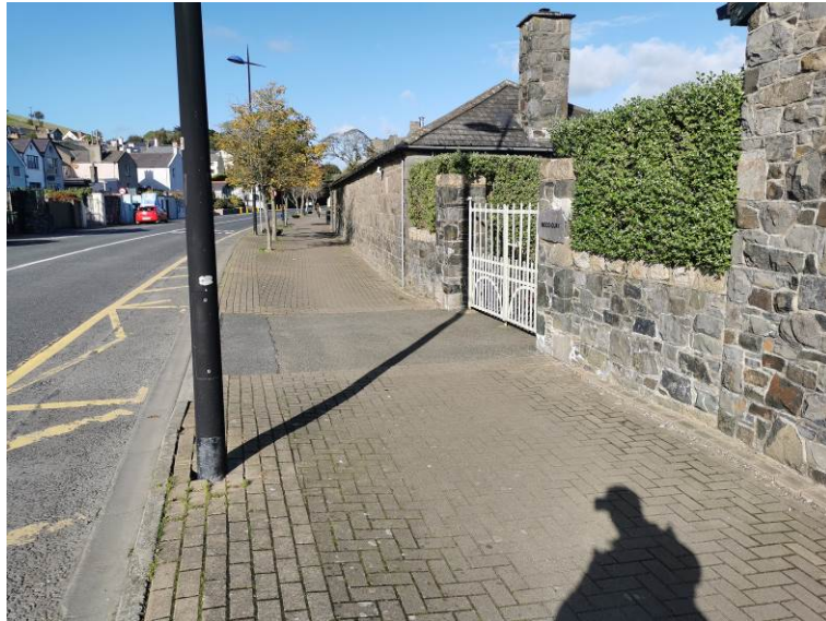
Plate 49 View of walls to CH33 Woods Quay, facing north
