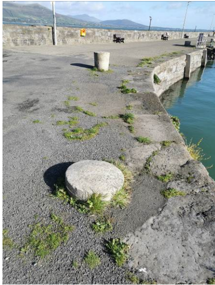
Plate 45 View of mooring posts to CH32, facing northeast
