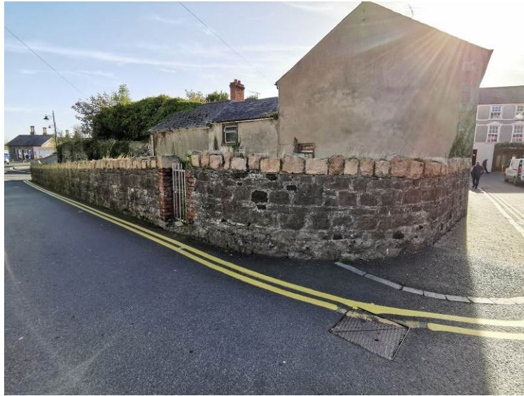
Plate 37 View of CH26, facing southeast
