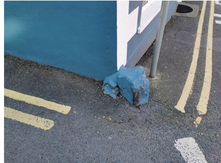
Plate 30 View of CH21, facing west
