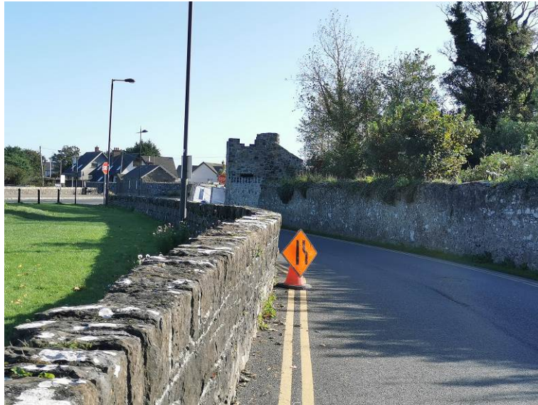
Plate 5 CH04 View of Sluice Gate Folly, facing southeast
