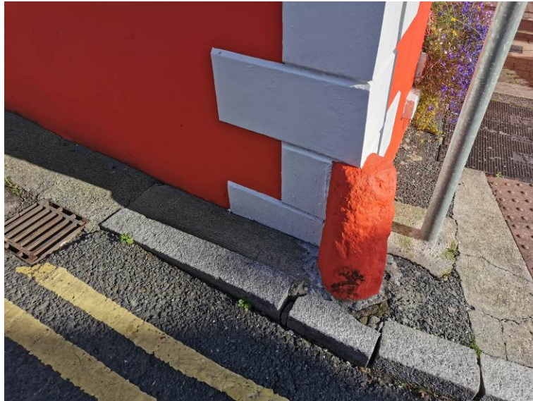
Plate 33 View of CH24, facing northeast
