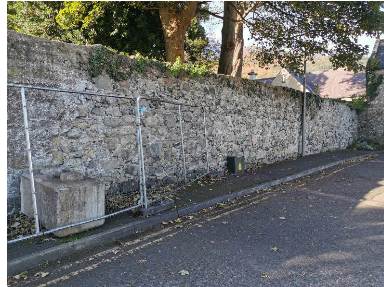
Plate 6 CH05, View of boundary wall, facing northwest
