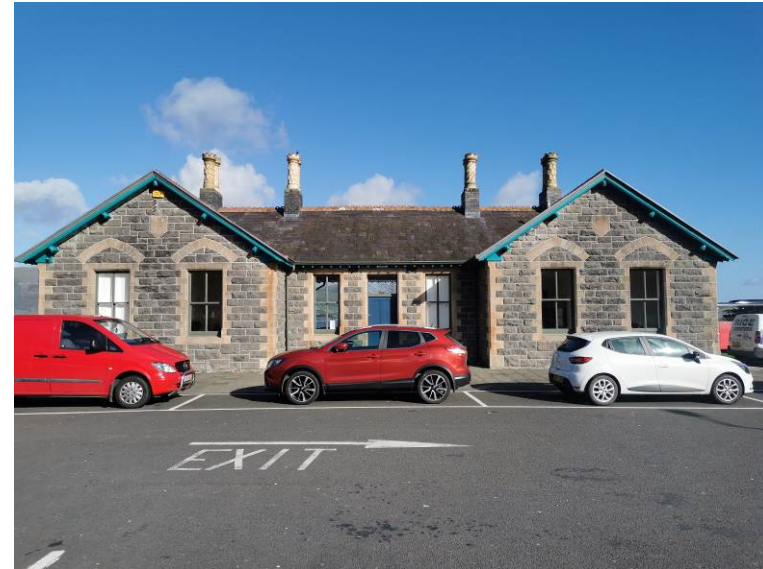
Plate 50 View of former railway station to CH34, facing east
