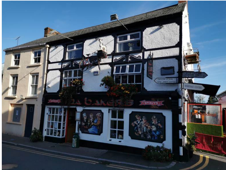
Plate 21 View of building to CH15, facing northeast
