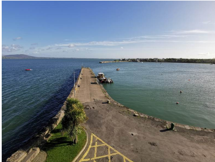
Plate 43 View of pier to CH32, facing east
