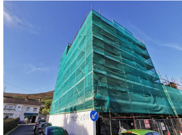
Plate 34 View of CH25, facing west
