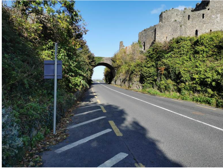
Plate 41 View of railway cutting CH30, facing northeast
