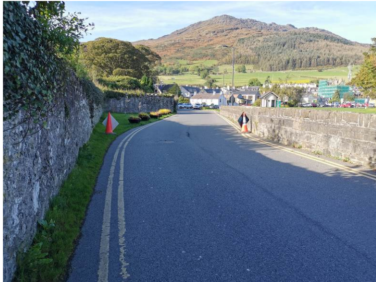
Plate 7 View of CH06 enclosing walls to Ghan House, facing west
