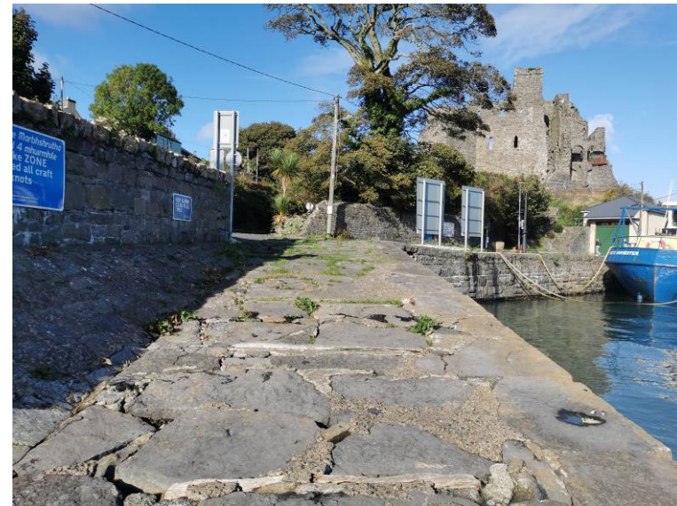
Plate 48 View of slipway to CH32, facing north
