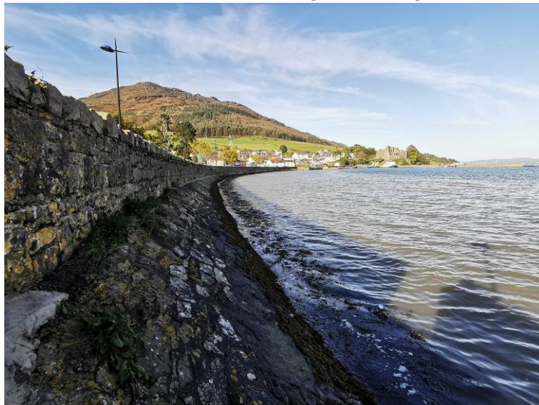
Plate 3 CH02 Sea wall, facing north
