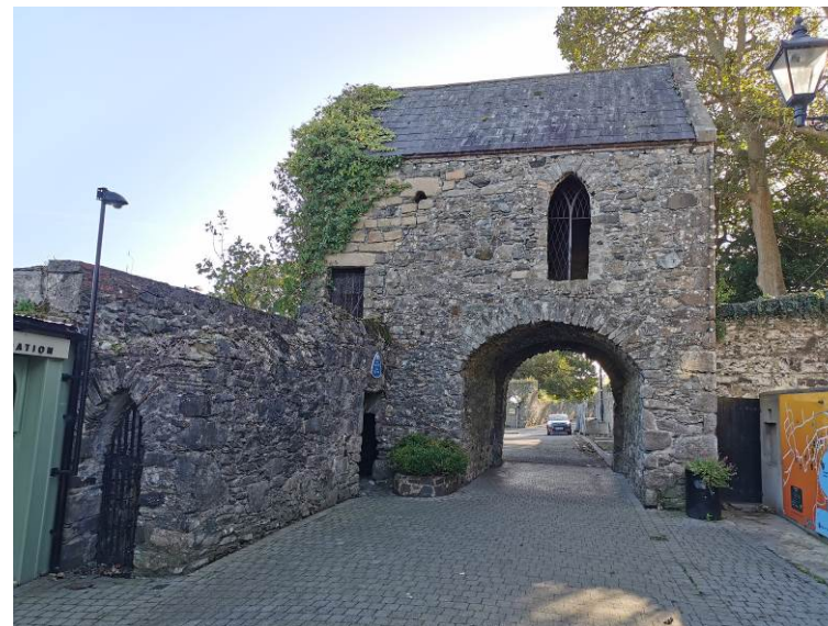
Plate 10 Interior view of CH07 The Tholsel, facing southeast
